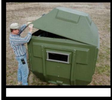
9. **ALL BOLTS IN THE WALLS AND ROOF MUST NOW BE TIGHTENED**
