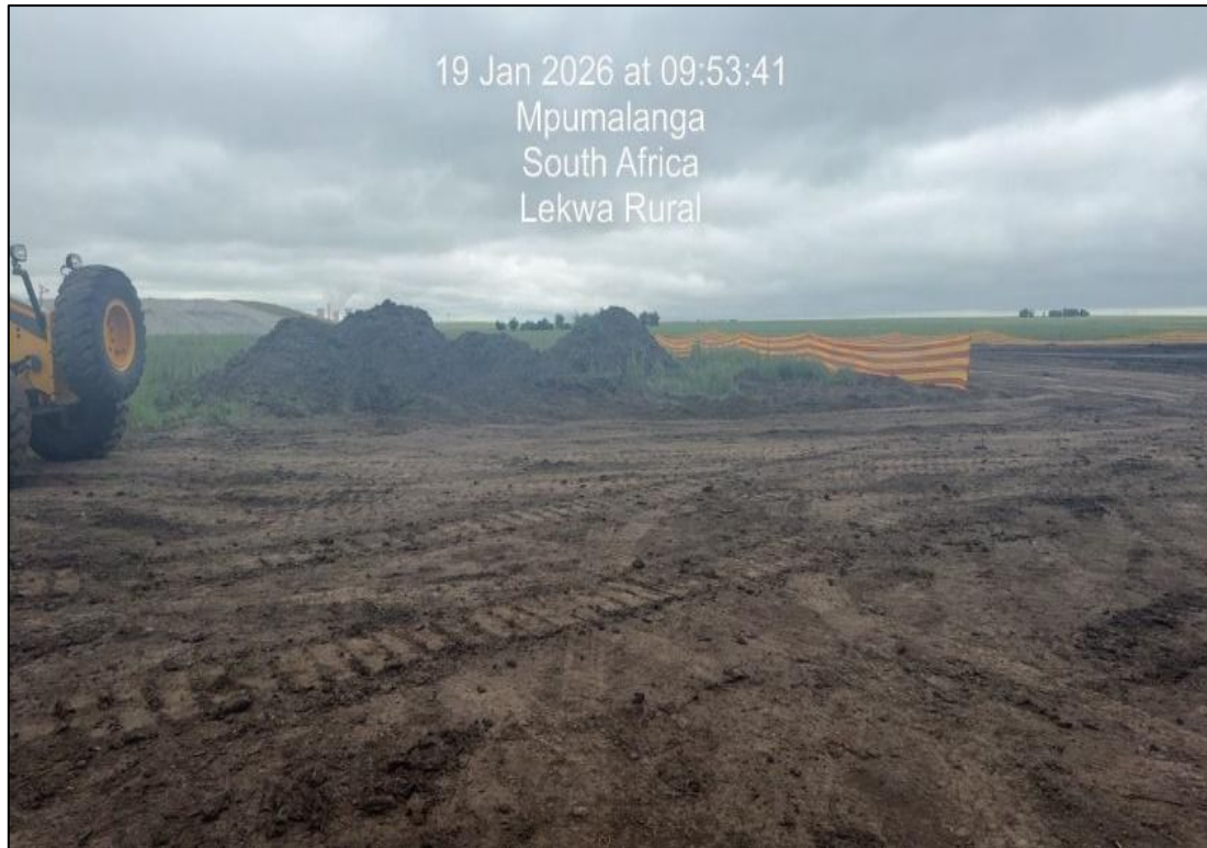
Figure 7: Stockpiles topsoil at the TSF.
