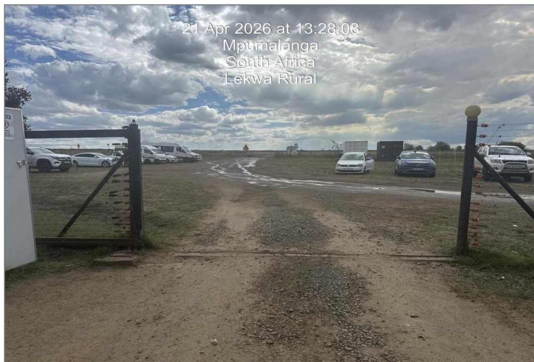
Figure 2: Dust supressing at the office area.
