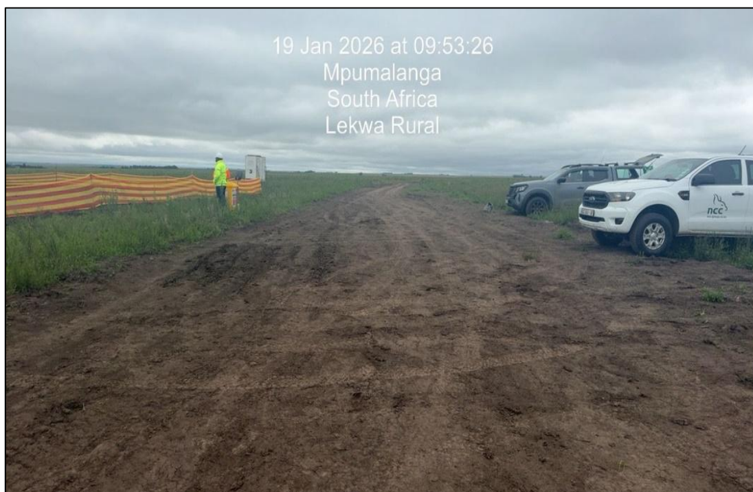
Figure 6: Access Road to the TSF area.
