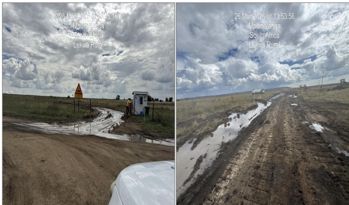
Figure 1: Condition of the access road
