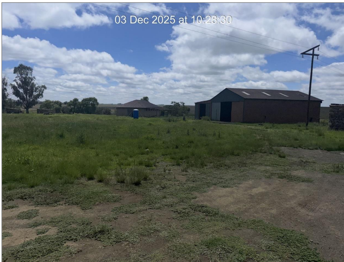
Figure 4: Building Structures onsite
