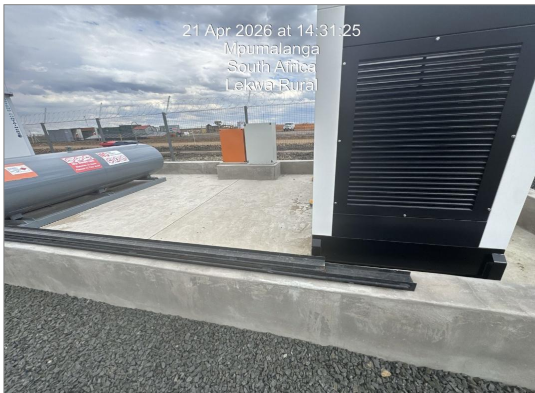
Figure 8: Diesel Bunt at the TSF area.
