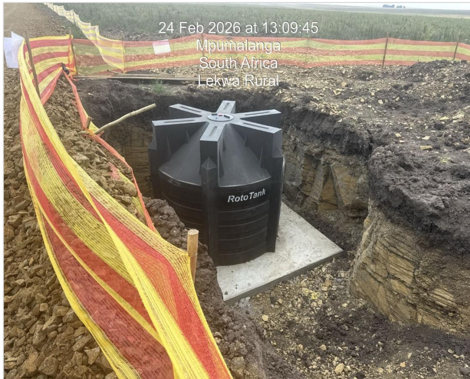
Figure 1: Conservancy tank under construction
