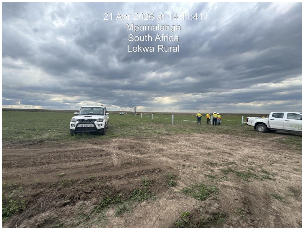
Figure 9: Pile installation at Tournee 2.
