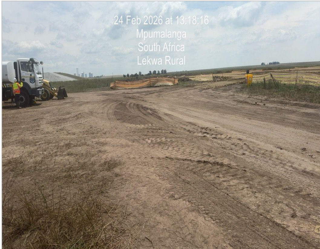
Figure 5: Dusty access road to the TSF area.
