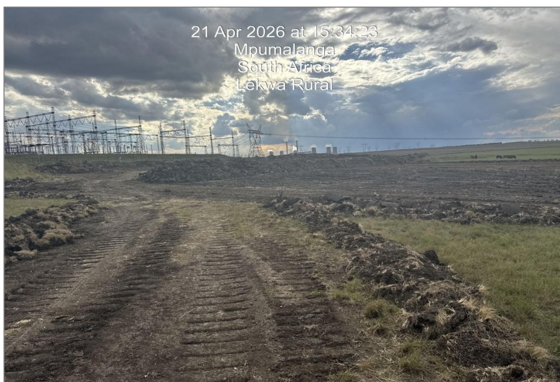
Figure 2: Clearing and grubbing at the substation.
