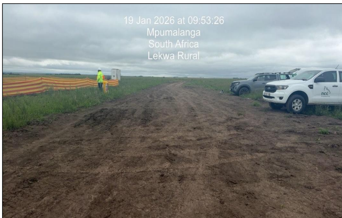
Figure 6: Access road to the TSF area.
