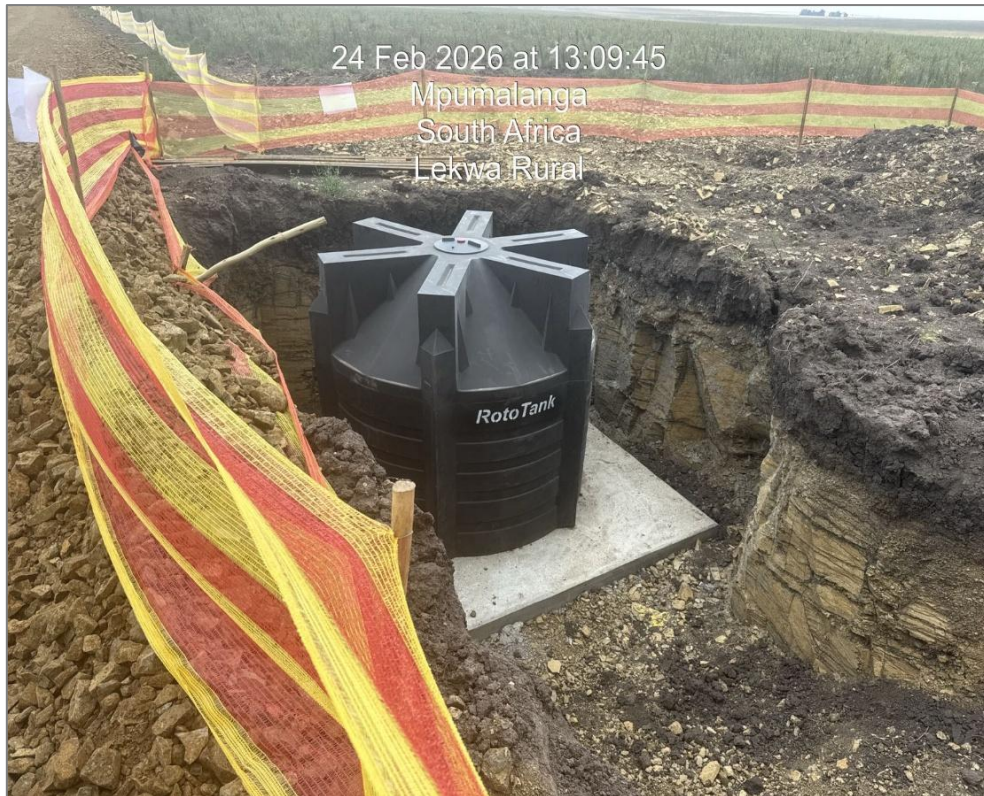
Figure 1: Conservancy tank under construction
