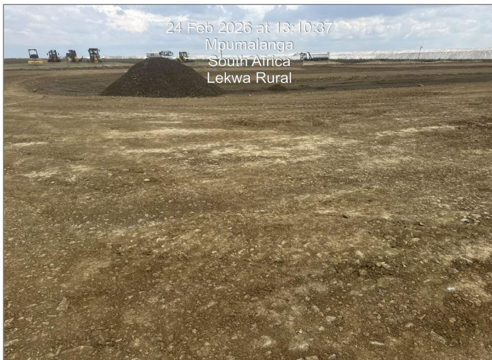
Figure 2: Compacted material at the TSF area
