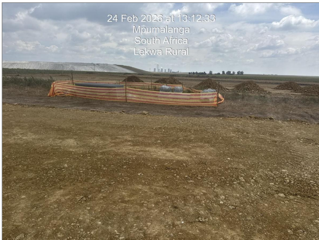
Figure 6: Stockpiles of Imported material to the TFS area.
