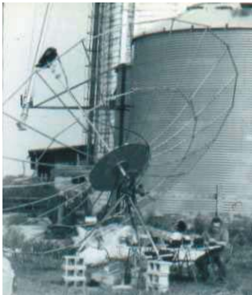
Figure 10 Portable 20' stress dish. a) Assembly, b) In operation, and c) Center hub
