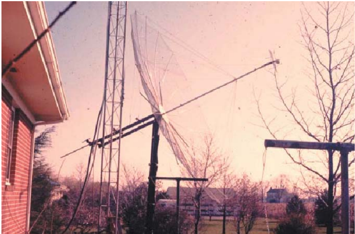
Figure 1 Twenty foot stress parabolic reflector used on 432 EME for many ears at K2UYH and later W3CCX
