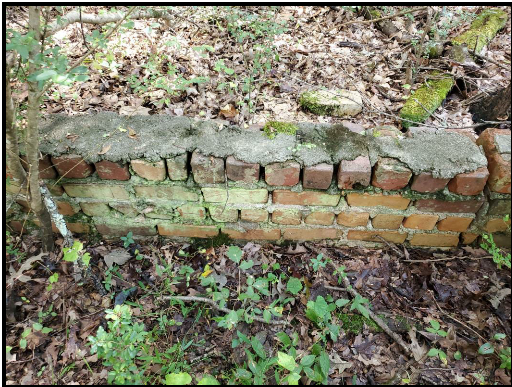
Figure 6.19. Brick Foundation
