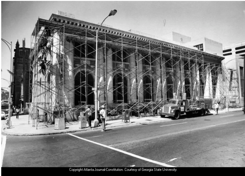
Figure 4.6. Dismantling of the Carnegie Library facade for construction of a new public library, 1977 https://digitalcollections.library.gsu.edu/digital/collection/ajc/id/11655/rec/71
