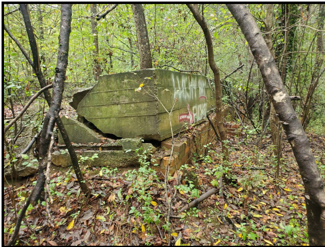
Figure 6.29 Remains of Brick and Concrete Block Foundation Structure
