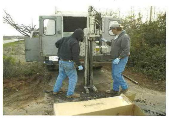
Photograph 2: View of the direct-push equipment advancing Soil Boring 1.
