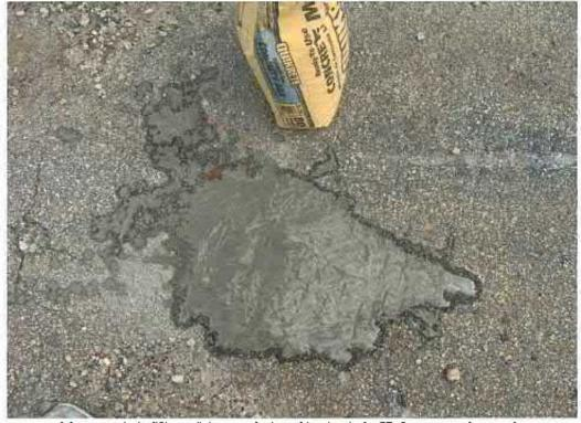
Photograph 4: View of decommissioned boring hole SB-2, cemented to grade.
