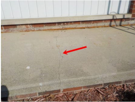
Cracked cap.
