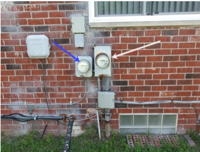
Main meter is white arrow. Blue is AC.
