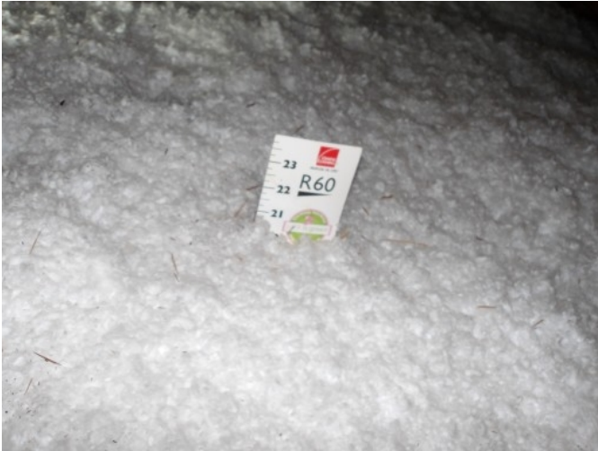
21 inches of blown in fiberglass insulation
