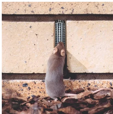
Example Picture - The mesh stops rodent and insect intrusion.
