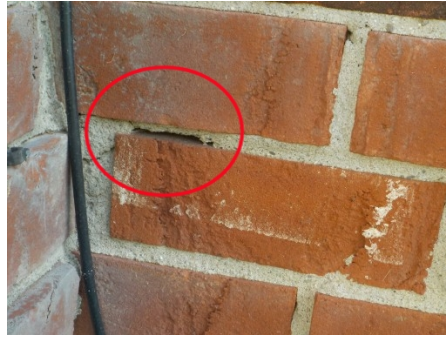
Fill any missing mortar to keep bricks supported
