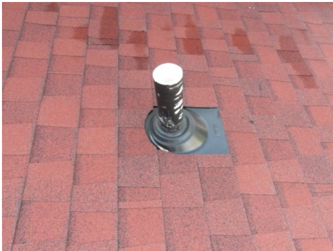
Through roof plumbing vents
