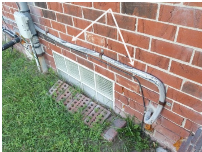
Service entrance wire sheathing is age deteriorated.
