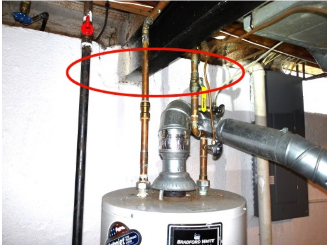
Bond water pipes and gas line.
