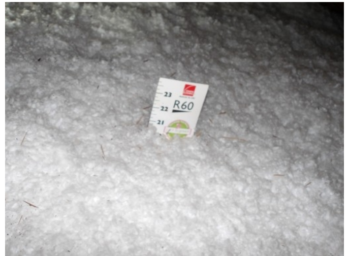
21 inches blown in insulation
