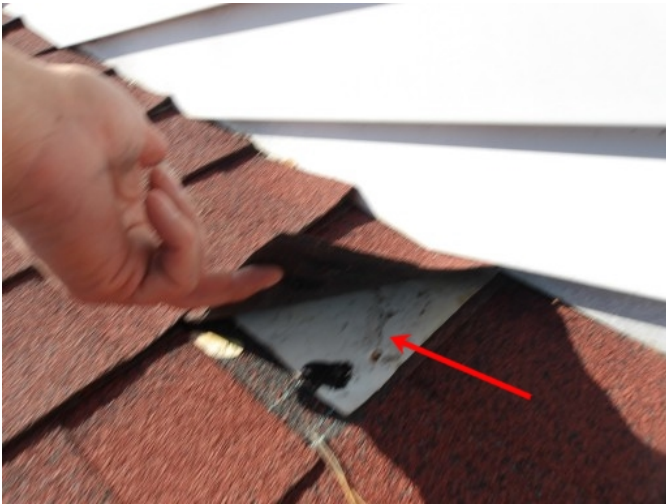
Step flashings are present at roof to wall transitions.
