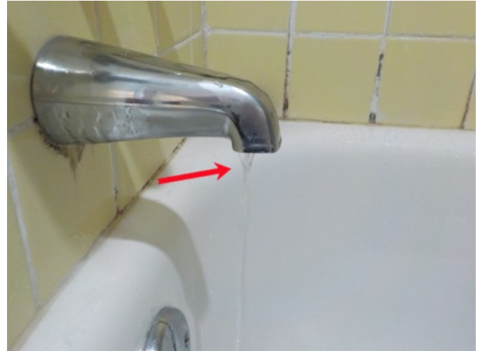
Not all water gets to showerhead - diverter works at about 80%
