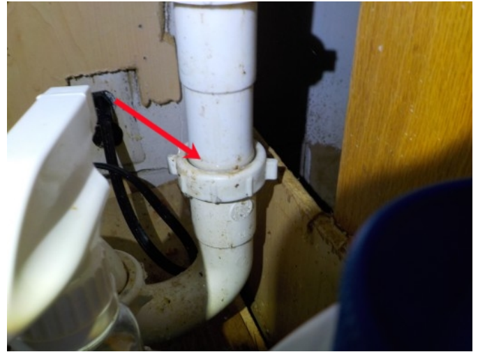
Leak detected.
