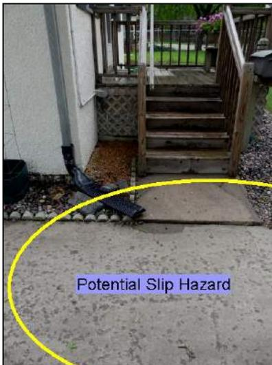
Downspout drains onto the walkway / driveway.
