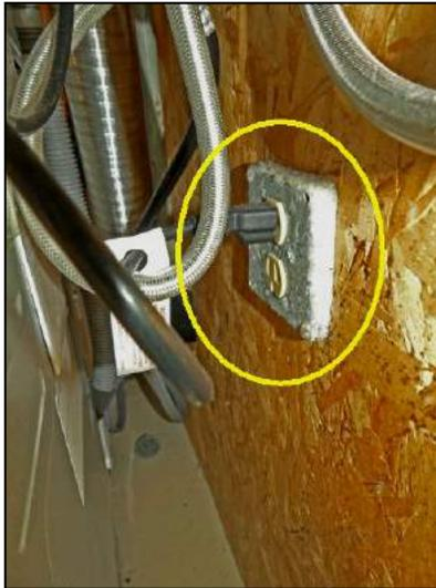
Wash Machine outlet is NOT GFCI protected.
