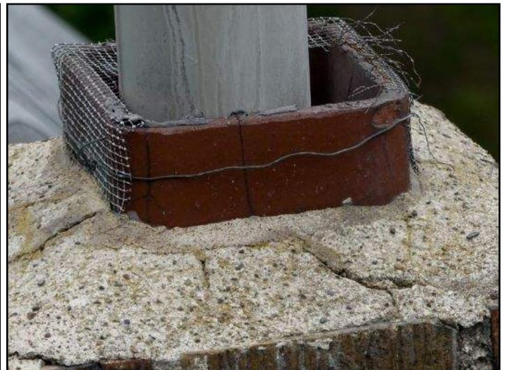
Wire mesh is damaged and missing.
