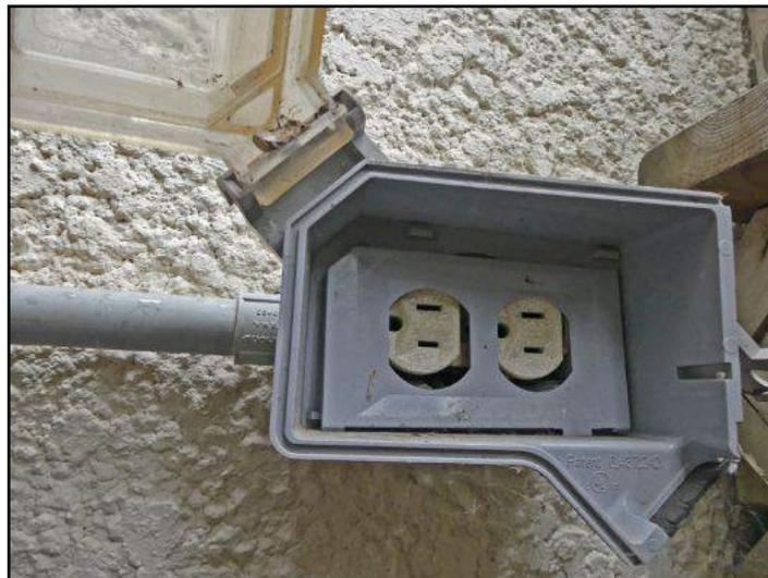
Exterior outlets on the house are not GFCI protected.
