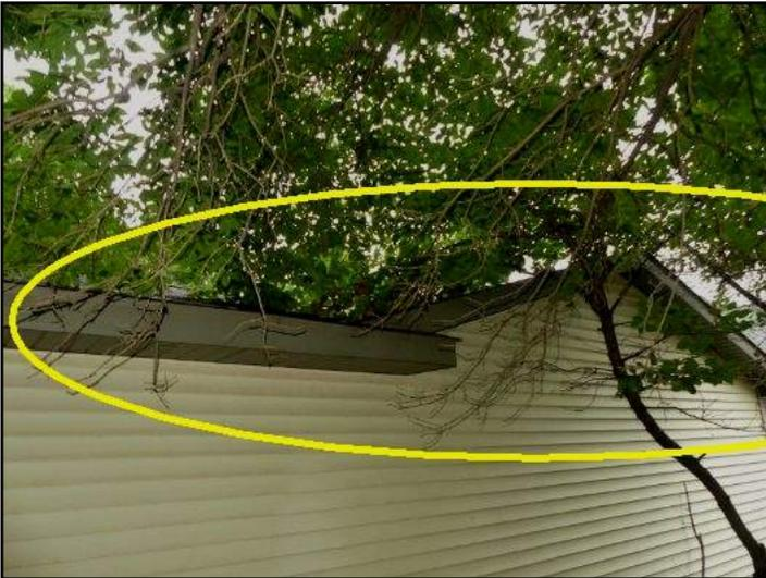
Tree branches are in direct contact with the Garage siding and roof.
