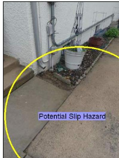
Gutter drains onto the walkway / driveway.
