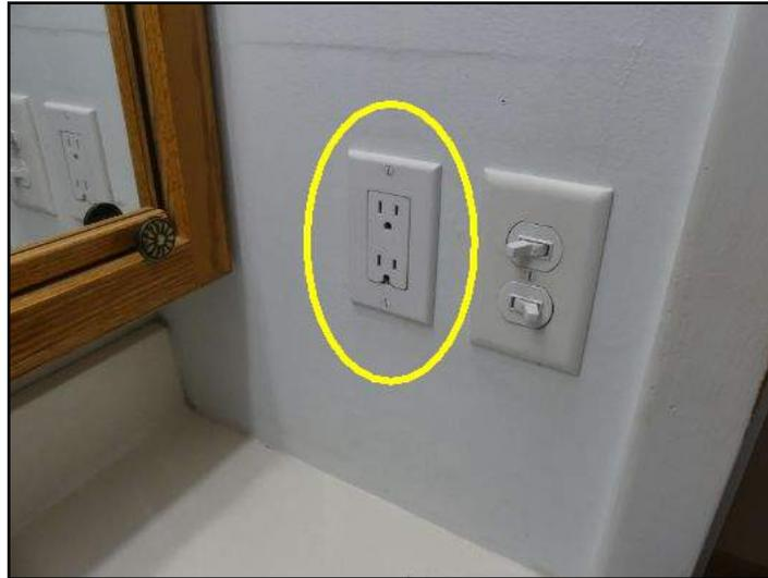
Outlets should be upgraded to GFCI for safety.
