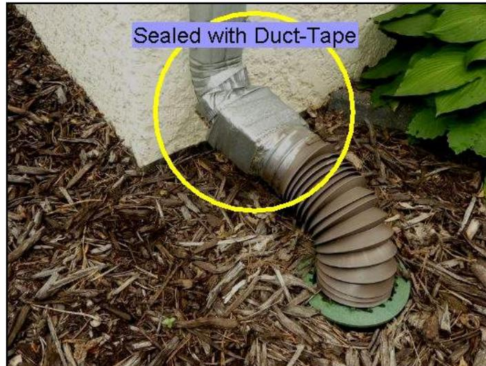
Gutters appear to drain into a buried drain tile.
