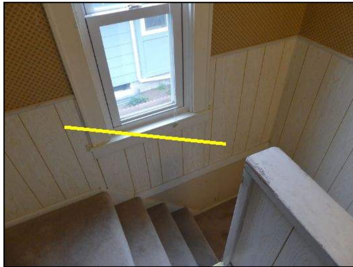
Handrail should be added for safety.
