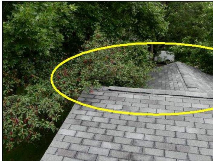
Branches are in direct contact with the structure / roof.
