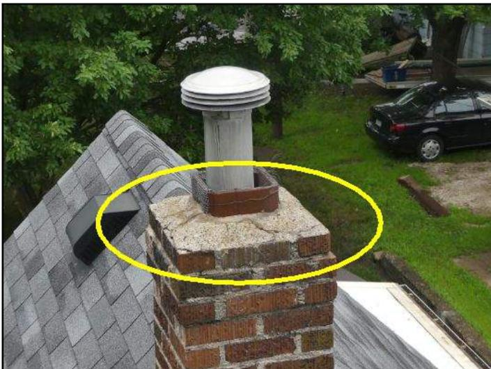
Concrete crown is cracked.
