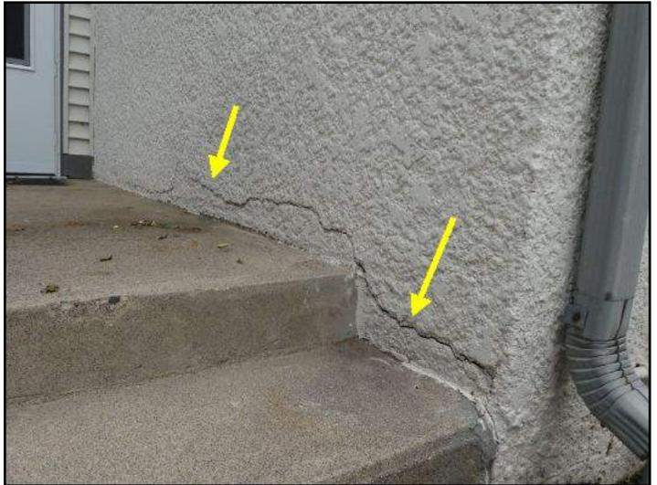
Cracking is noted in the Stucco.
