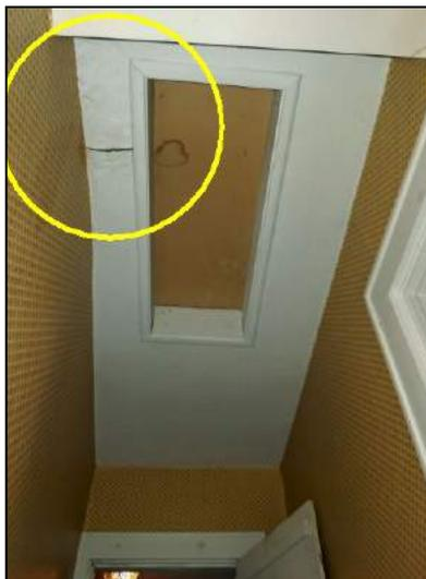
Water staining and damage is noted.
