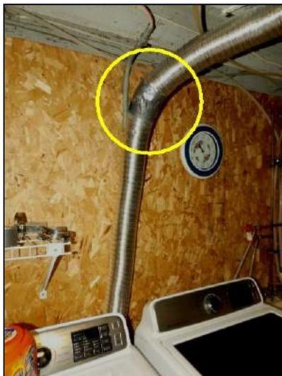
Improperly sealed with flammable Duct-Tape.
