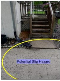
Downspout drains onto the walkway / driveway.
