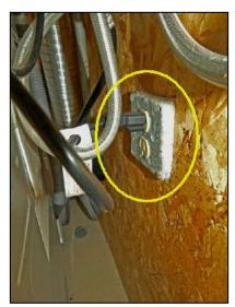
Wash Machine outlet is NOT GFCI protected.
