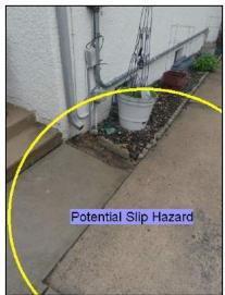
Gutter drains onto the walkway / driveway.
