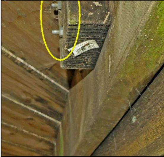
Handrail posts are through bolted to the joists.
