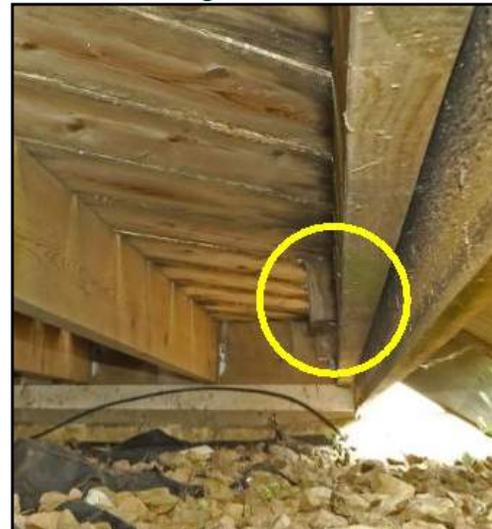
Handrail posts are fastened to the joists.
