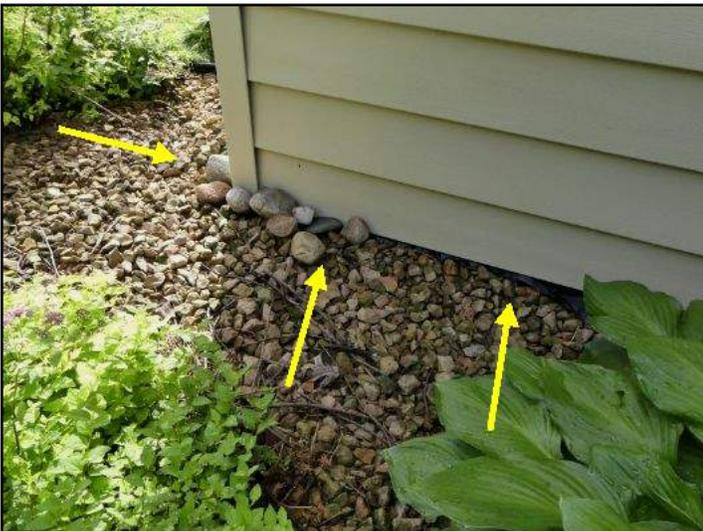
Siding should not be in direct contact with ground.
