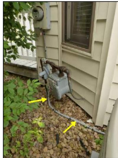
Armored cable to the A/C is not properly attached to the structure.
