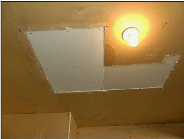
Firewalls ceiling are not taped and sealed.
