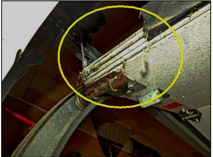
Bottom weatherstripping should be replaced.
