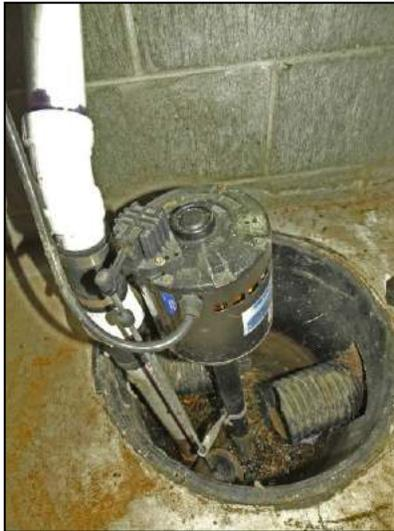
A cover should be installed for safety.
