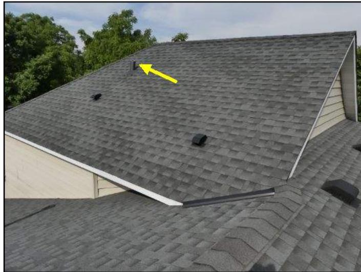
Vent stack with poorly fitting lead ring.
