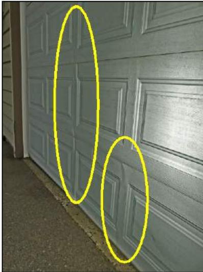
Bottom three sections are damaged.
