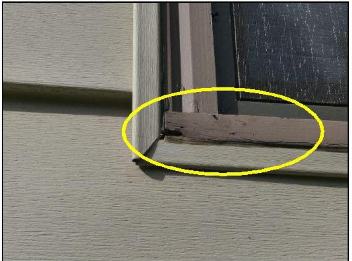
Deterioration at the exterior wood frame.
