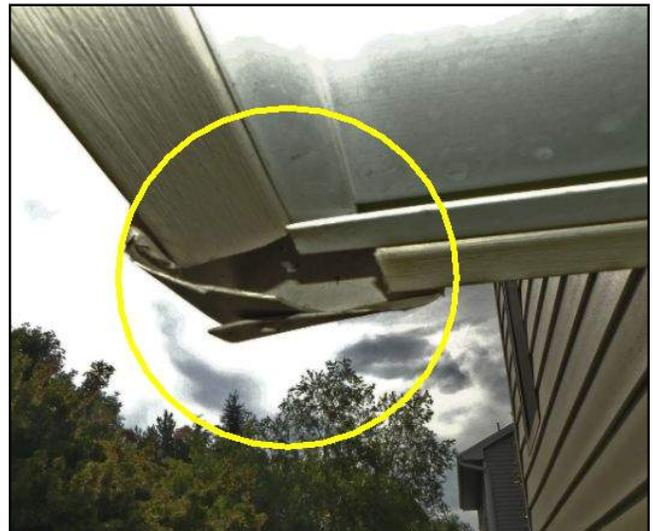
Gaps at the bottom of the corner trim. It is not properly secured.
