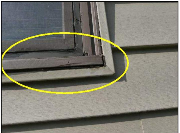
Deterioration noted at the exterior window frame.
