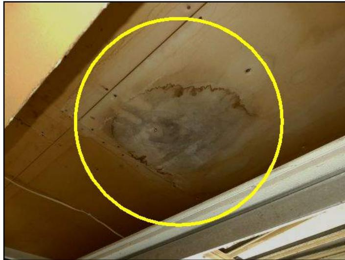
Water staining is noted. It tested dry at the time of inspection. Monitor.
