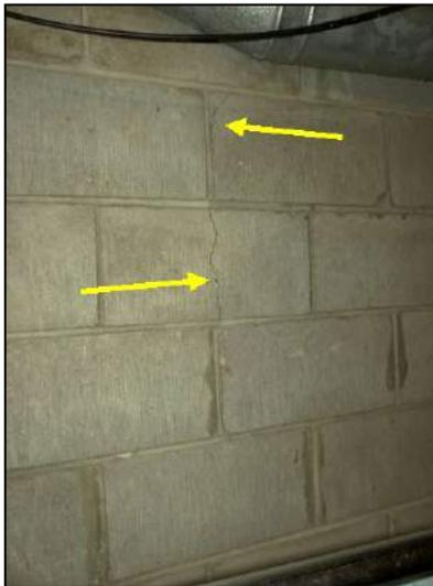
Normal settlement cracks are noted in the block walls.
