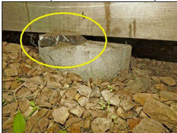
Beams and joist are not properly supported.
