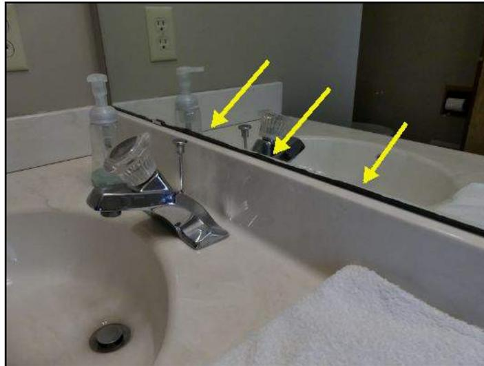
Minor deterioration is noted along the bottom edge of the mirror.
