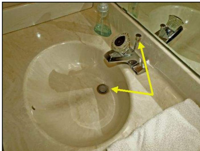
Drain diverter does not function.
