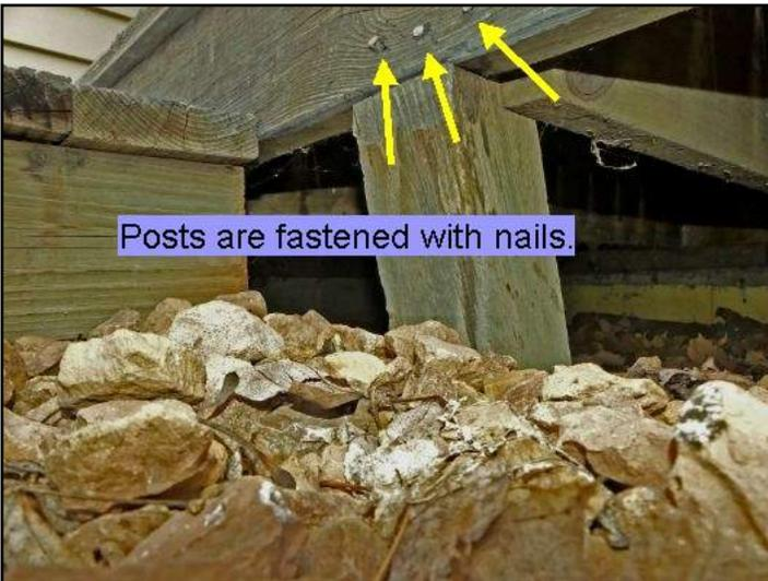
4" x 4" support posts are not properly fastened to the beam.
