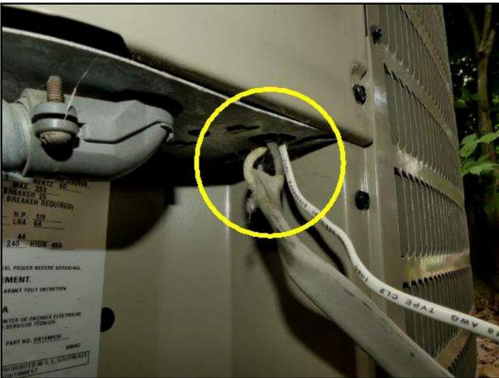
220V electrical wire is not properly connected.
