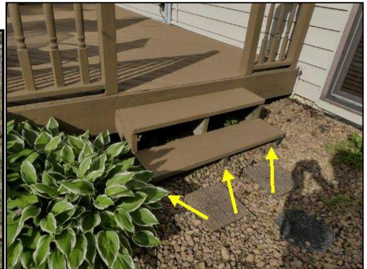
Stair stringers are in direct contact with the ground.
