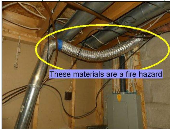
Dryer vent should be repaired with proper materials for fire safety.
