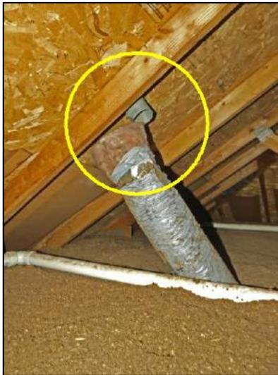
The exhaust vent for the Master Bathroom is not attached to the roof vent.
