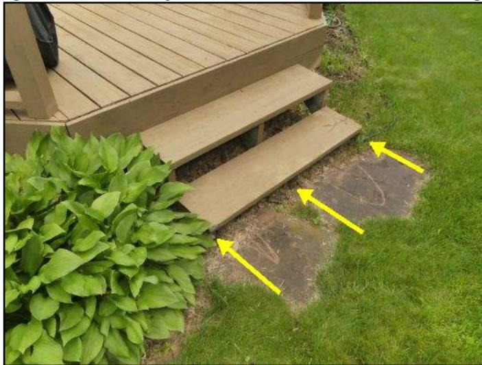
Stair pad at the front of the Deck is in direct contact with the ground.
