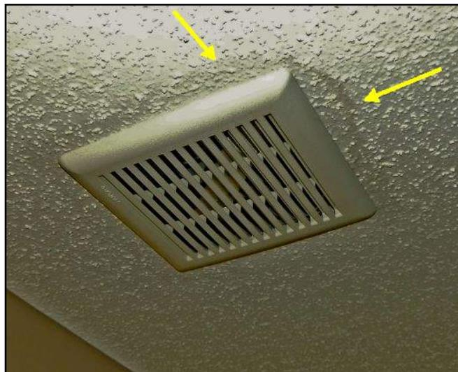
Water staining is noted around the exhaust fan.
