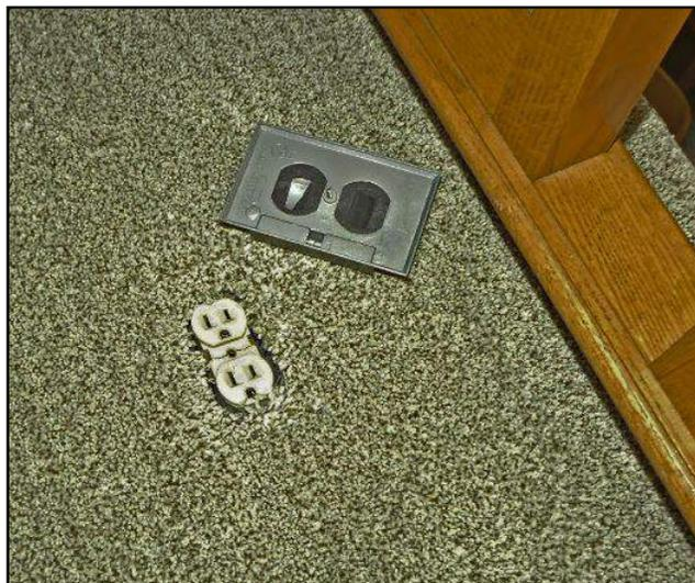
Floor outlet is broken, the cover is not secured in place.
