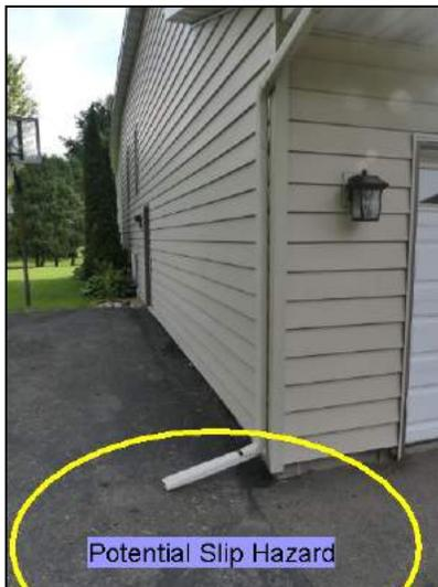
Downspout drains onto the driveway / walkway.
