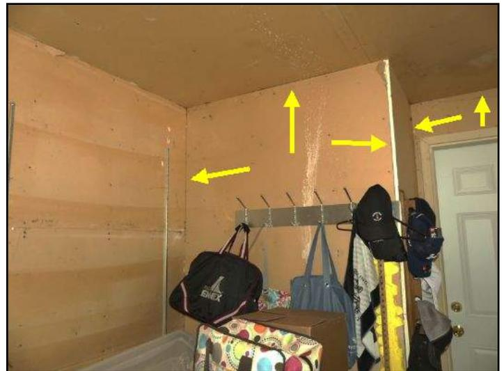
Firewalls are not taped and sealed.
