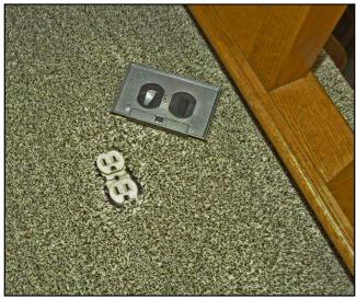
Floor outlet is broken, the cover is not secured in place.
