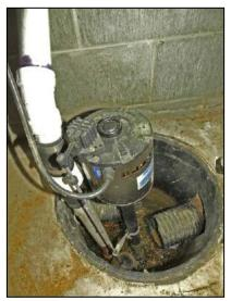
A cover should be installed for safety.
