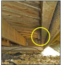
Handrail posts are fastened to the joists.
