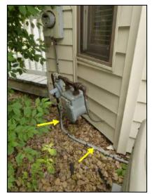
220V electrical wire is not properly connected. Armored cable to the A/C is not properly attached to the structure.
