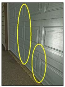
Bottom three sections are damaged.
