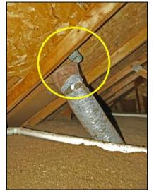
The exhaust vent for the Master Bathroom is not attached to the roof vent.
