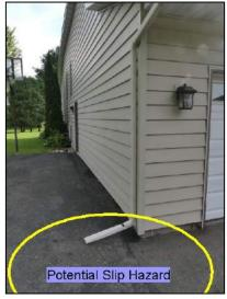
Downspout drains onto the driveway / walkway.
