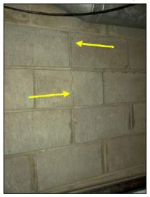
Normal settlement cracks are noted in the block walls.
