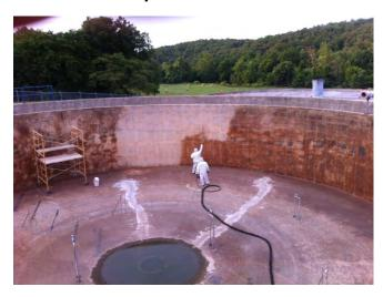
In the Spring of 2013, the City of Harrison was nearing completion of the Phase 1 WWTP Improvements, which included the conversion of two abandoned clarifiers to aerobic digesters. When the contractor began filling the aerobic digesters for testing, it was determined that the concrete tanks leaked.
