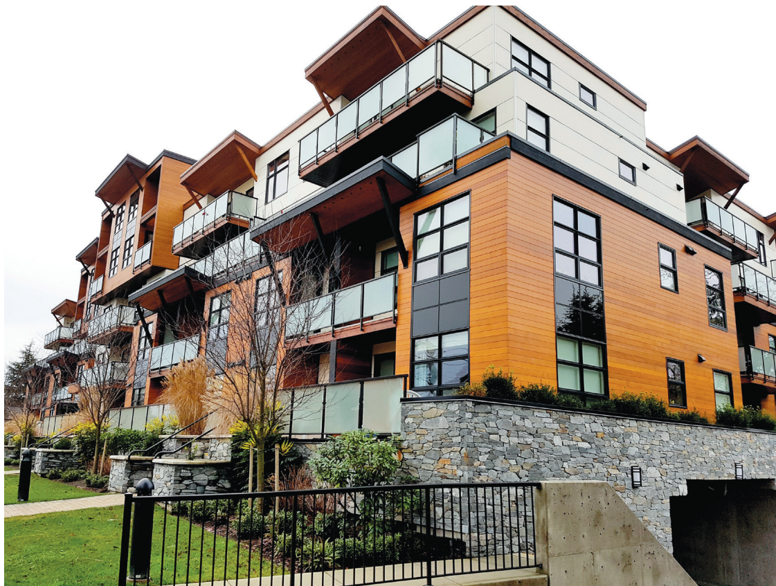
Villa Plumbing And Heating has had a tremendous amount of experience working on large scale condo projects
