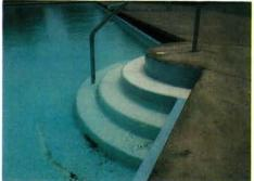
Steps—State codes require that steps be in a contrasting color. In addition, all steps, ledges, and laminated decks are skid proofed.
