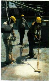
90% of the "P.I.P." pool stress material is installed with the spray-up technique. All materials are installed from 1/8"-1/2" thick (concrete), 1/32"-3/16" thick over metals in a neutral color to insure maximum visual inspection. All laminate is rolled to insure complete resin coverage. (Above)
