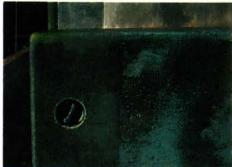
Pool inlets, drains, lights, etc; are thoroughly cleaned to remove overspray of resins, fibers and gel coats. If taped, tape is removed and tape residue is removed. This picture also shows a section of fiberglass laminate against the concrete surface.
