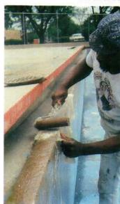
Hand lay-up—The use of the hand lay-up technique is often used in the areas that require close detail work. Hand lay-up allows for more application control to avoid overspray of resins and fibers onto areas that will not be laminated.
