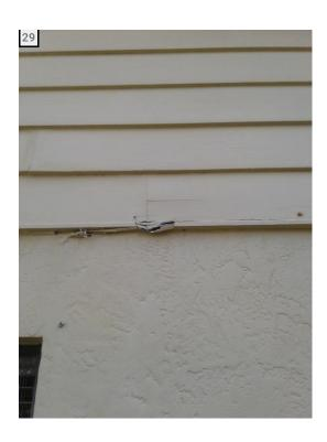
Wood under flashing missing
