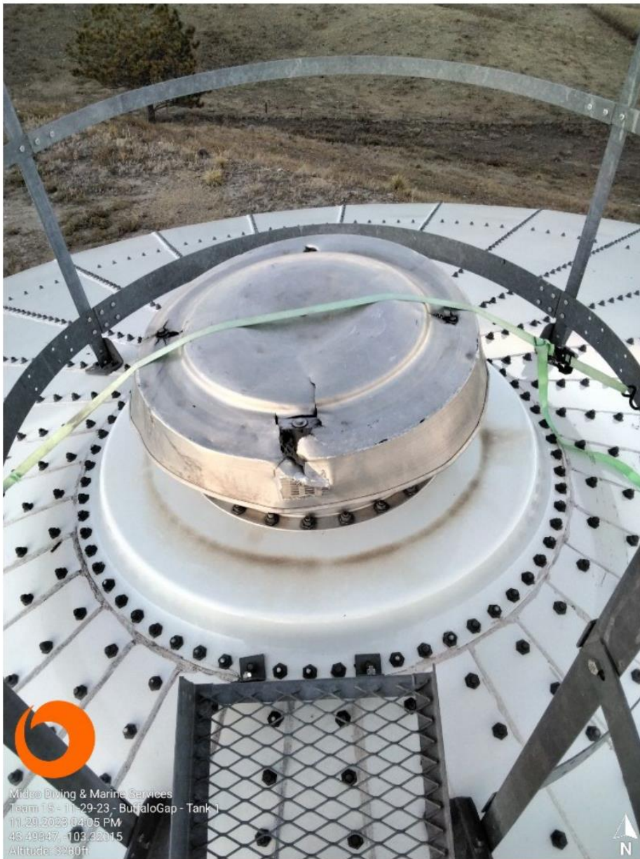
ISSUE # 2 (ABOVE GRADE) ROOF VENT DAMAGE
