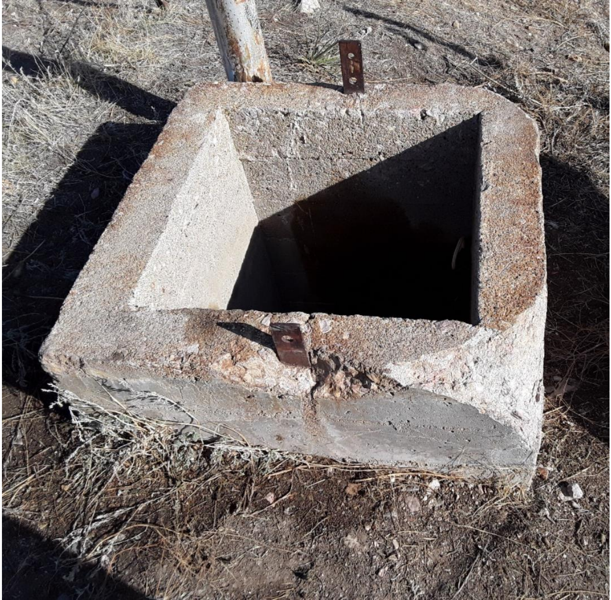
ISSUE # 1 (BELOW GRADE) ACCESS HATCH WITH SPALLING
