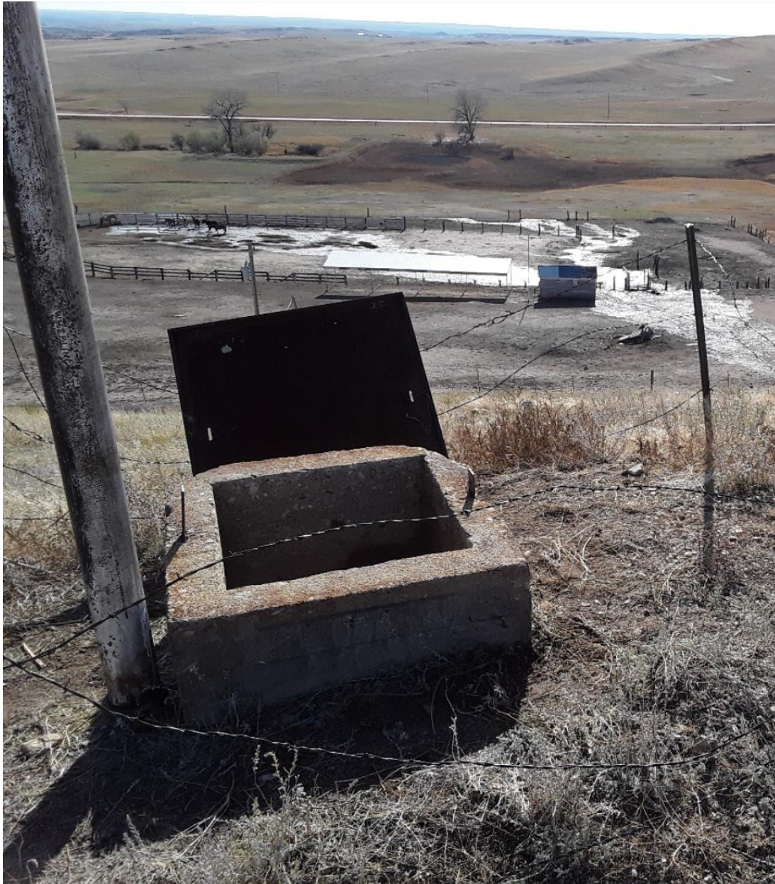
ISSUE # 1 (BELOW GRADE) ACCESS HATCH WITH METAL TOP REMOVED
