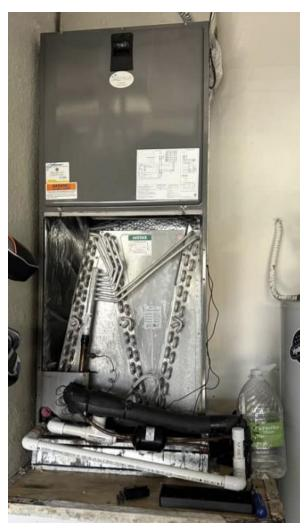
This system is an "N" configuration with one coil on the left side which dispenses into one drain trough, and the other two coils form a "V" and share a common drain trough.
