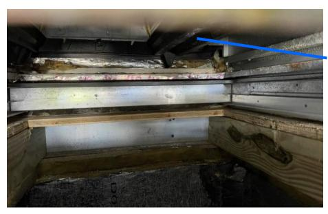
After placement, the filter opening provided visual access from underneath the system that the nozzle and dispense tube were secure in the drain trough and had not popped out while being inserted.
