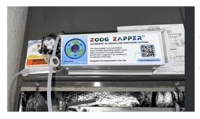
The Reservoir Holder was mounted on the upper cabinet to provide clearance in case the lower cabinet panel had to be removed in the future. The customer preferred the system being elevated.
