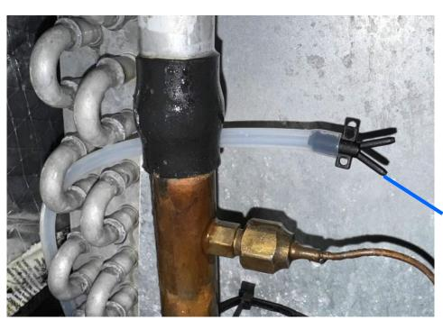
The dispense tubing was threaded through the coil aluminum tubes to anchor the dispense tubing, and the dispense tubing is brought to the center of the unit.
