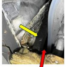
The left coil dispense tube was placed on top of the left coil. The placement wire was used to reach all the way to the back of the drain pan. The drain pan (yellow arrow) had a height side wall of about 2.5" which is perfect for placement of the Single-Port Nozzle (red arrow):
