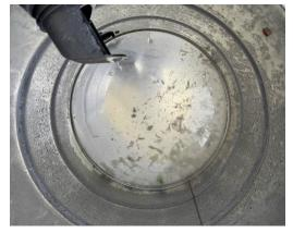
Vacuuming out the drain line – there was bacteria in a quantity that was surprising based on the drain line just being cleaned out a few weeks ago.
