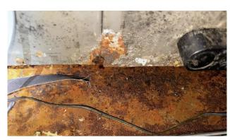
The sides of the panels have excessive rust.
