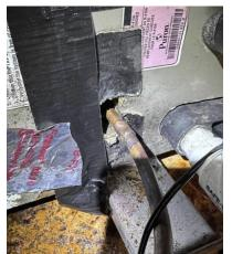
The entry point of the dispense tubing was the standard oval opening with the rubber plug, except there was no rubber plug – just a hole.
