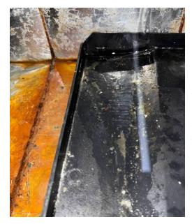
Looking to the left of the drain pan, the floor of the unit has standing water, about 1/4" deep.
