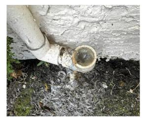
Vacuumed the drain line. Since this is an attic installation there was only a small amount of condensate due to the slope of the attic drainpipe, then a vertical drop from the attic down to the exit port. There was some Zoogloea at the exit port couplings and some Zoog visible on the ground.
