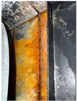
My assumption is that the pitch of the drain pan/cabinet is incorrect, and water is <u>overflowing</u> the left back corner of the drain pan and spilling down to the floor of the cabinet.
