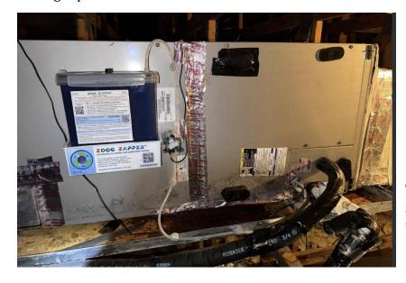
The dispense tubing was routed along the secondary drain pan using the magnetic tube holders.
