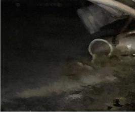
This unit has a tube from the coil connection plate down to the drain pan, and there was Zoogloea growing at the exit of the tube.
