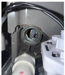
The tube was lowered down to the hole (left picture) and the tube is pulled out with a needle-nose pliers (center picture). The tube is attached to the Combo fitting on the threaded side of the fitting. (right picture)
