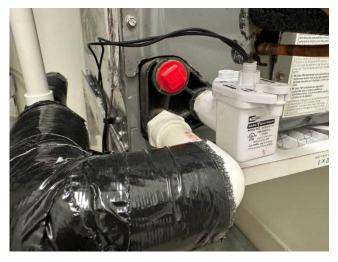
The entry point for the tubing will be the spare drain port (on both systems).
