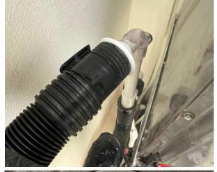
I put the vent tube back on and vacuumed out the drain piping.
