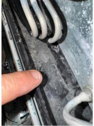
This system also had a "clump" of bacteria growing at the drain outlet. Eventually the drain port would have clogged.
