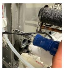
The stationary panel was loosened to have more access to lower the 380MM (15") tube down behind the stationary panel to line up with the outlet hole.
