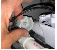
The combo fitting is inserted into the drain outlet hole.
