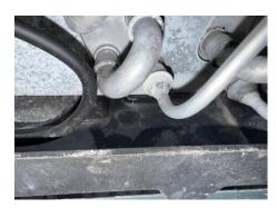
A Single-Port Nozzle is also going to be used on the right-side coils. The placement location could be placed in either of two locations, under the coil directly in the trough (left) or on the top of the coils (right) down inside the "V" at the far back.
