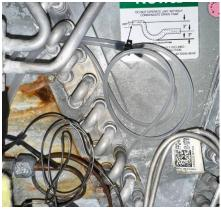
The 4mm dispense tube was threaded through the coils using the needle-nose pliers (easier with a pliers) and then the tube was connected to the Two-Port Manifold.
