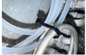
Wire ties were used to loosely hold the Two-Port Manifold to the tubing and to secure the dispense tubes to the coils.
