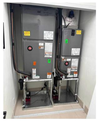
These systems clogged over the years, and I installed a Zoog Zapper on both. A few months later the homeowner decided to move the AC systems out of the attic because of all the previous problems. I went back to re-install both Zoog Zappers. Both AC systems were installed vertically and both systems required condensate pumps as a pump is the only way to expel the condensate.
