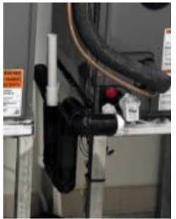
The trap is necessary for the condensate to exit the drain pan, the vent pipe provides air flow to allow the condensate to flow unimpeded to the pump.
