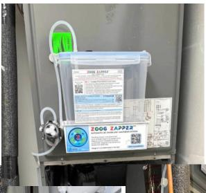
Next, the Zoog Zapper was placed on the upper panel, left side, because this is the side the copper tubing enters the cabinet.
