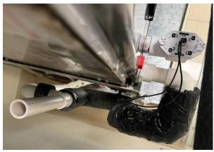
The PVC piping on both systems could be removed to be cleaned (good), and to be able to pull out the condensate pumps for cleaning and servicing.
