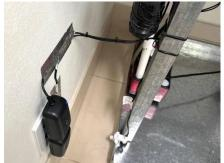
Aluminum tape was used to secure the wiring to the wall, and both aluminum tape and wire ties were used to secure the two power cables routed up to both pumps. The two cables were threaded through the two support frames to the pumps.
