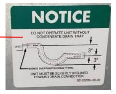
There is no trap, even though there is a label on the unit stating not to run the system without a trap.
