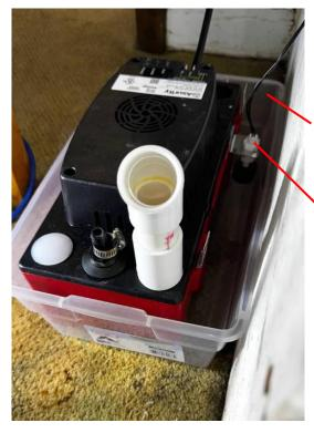
A plastic container was used to house the pump, so if there is a future pump failure water will be held in the container.
