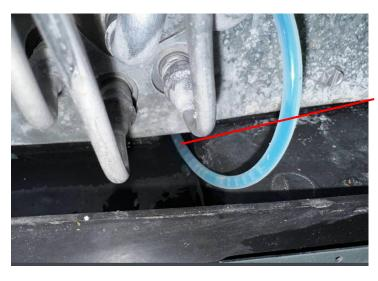
For the right-side drain trough dispensing, the Single-Port Nozzle was inserted into the drain trough directly using the placement wire.
