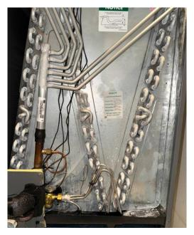
For the left drain trough dispensing, the Single-Port Nozzle was placed onto the top side of the coil using the placement wire to reach the far-back corner.
