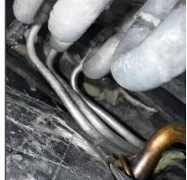
When this system clogged, the clog was most likely always in the drain line.
