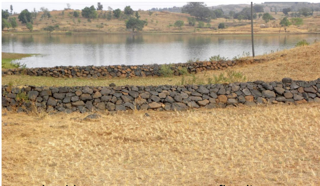
Loose boulder structure to prevent flooding, Nashik, Maharashtra, Feb 2014 | Sudha Narayanan
