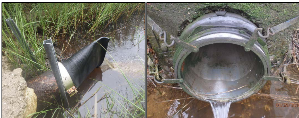
Figure 22. Examples of Functioning Backflow Prevention Devices Currently Installed. (left: recurved duckbill valve, right: WaStop® Inline Check Valve)
