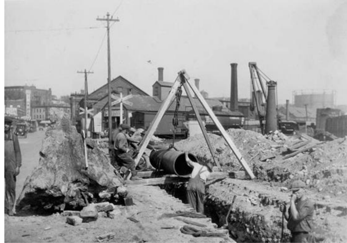
FGE 24-inch cast iron pipe installation - 1924
