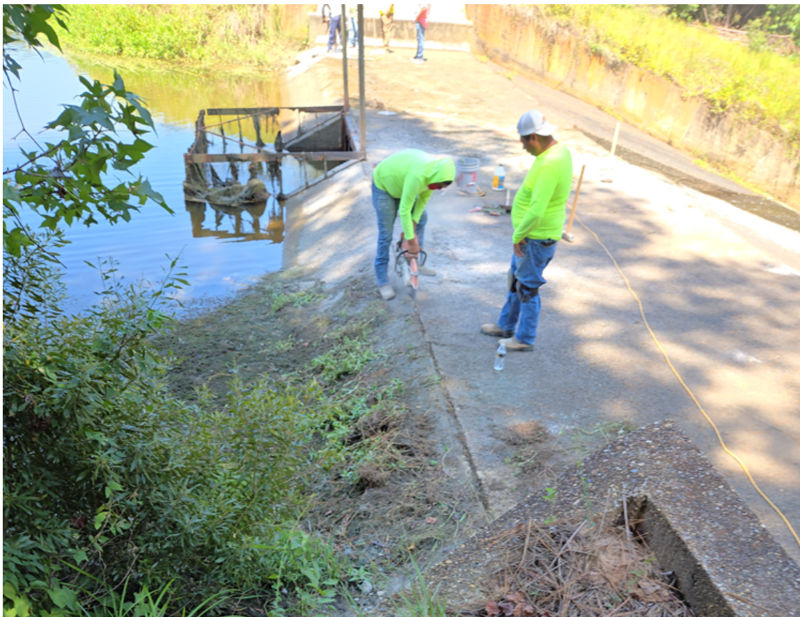
Figure 9 – Prepping the gaps in the spillway
