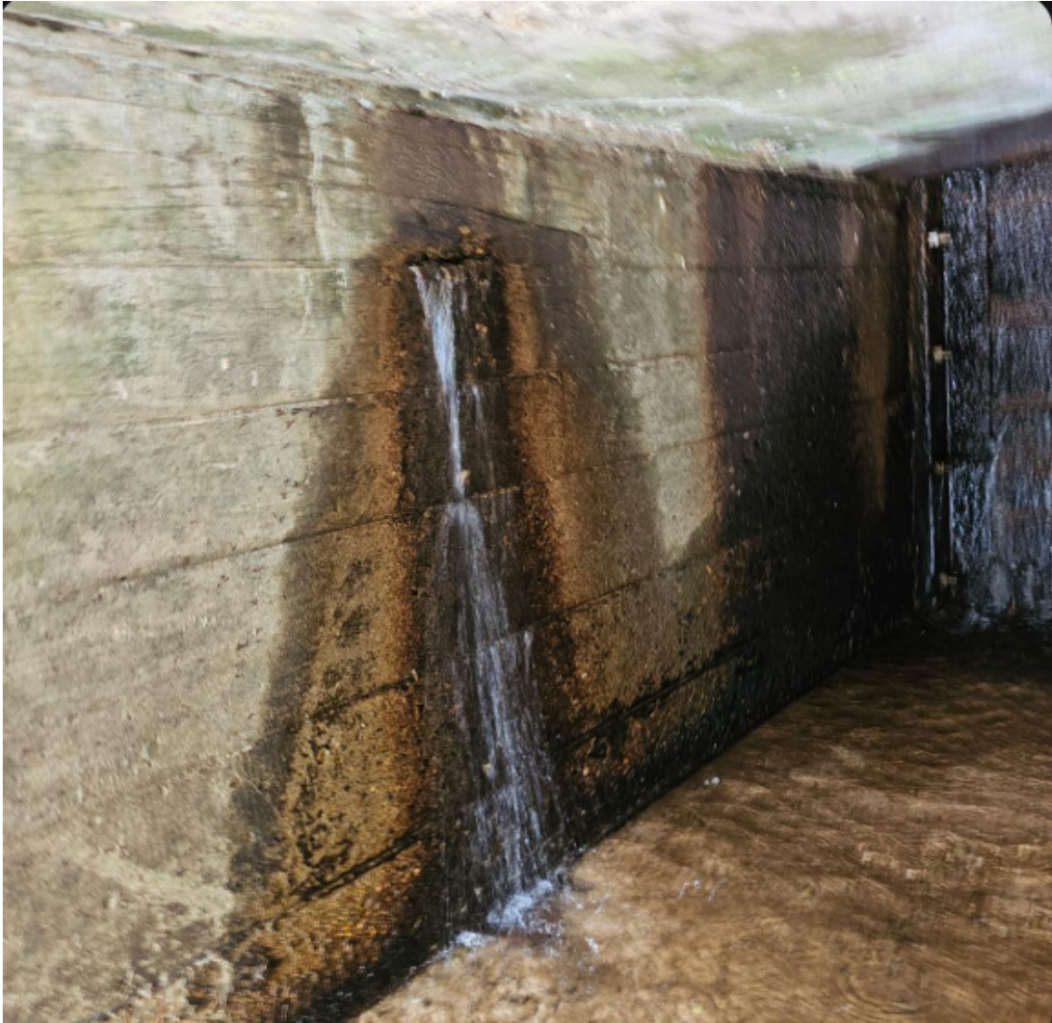
Figure 1 – Water leaking out of the spillway
