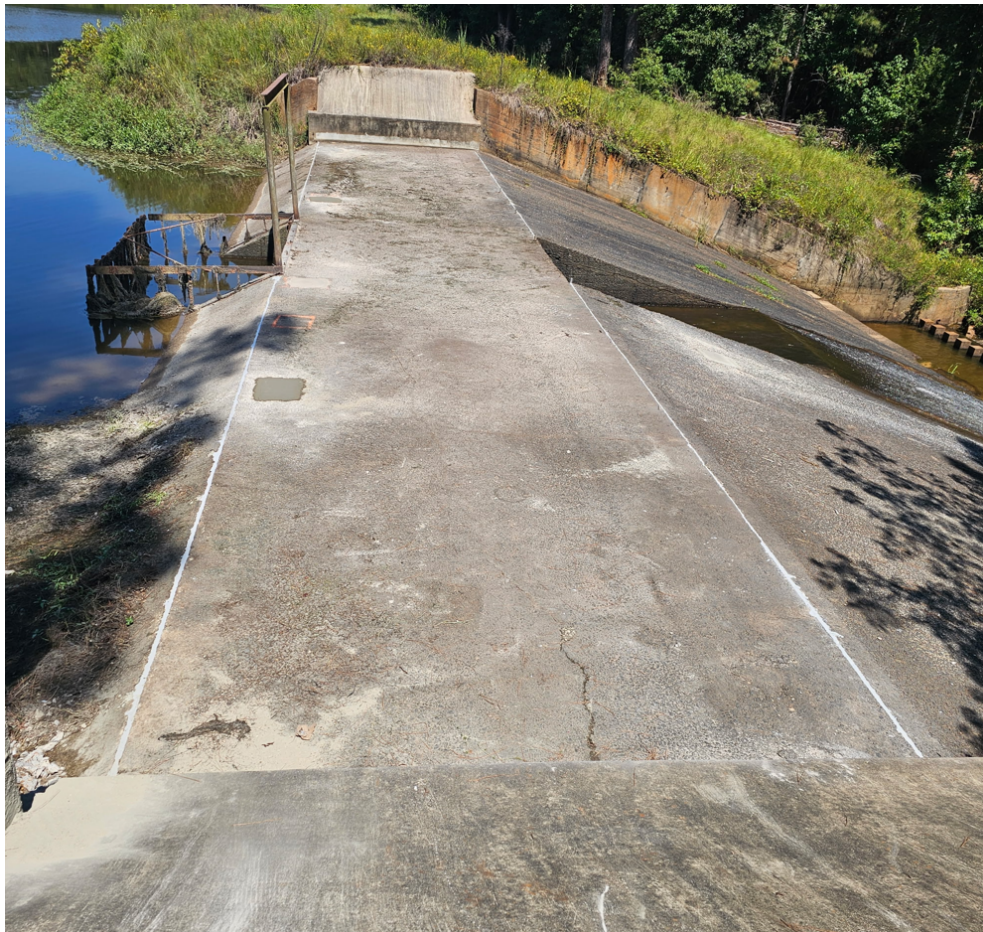
Figure 11 – Gaps in the spillway sealed
