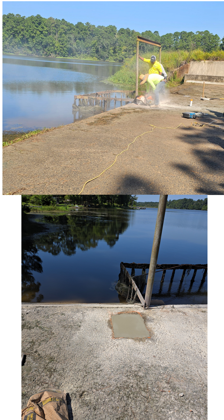
Figure 2 – Location of the first hole that was cut out
