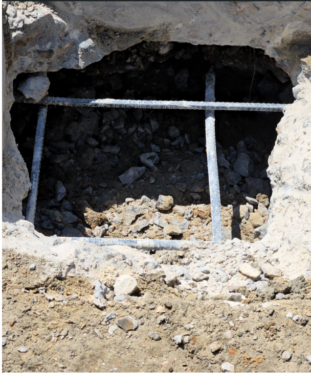
Figure 6 – Zoom in picture of the erosion on the North side of the spillway.
