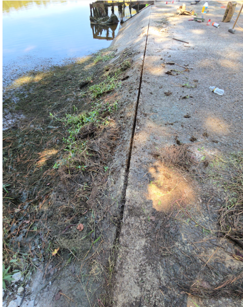
Figure 3 – Gap in the dam
