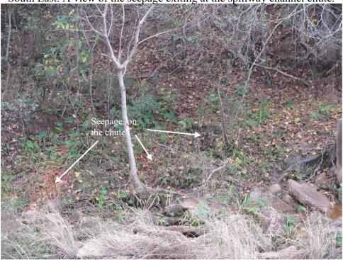
Photograph No. 48 – Closer view of the seepage exiting at the spillway downstream channel chute.
