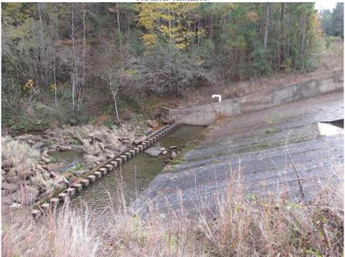
Photograph No. 40 – A view of the left 4-inch diameter pipe installed as a part of the spillway drain system.
