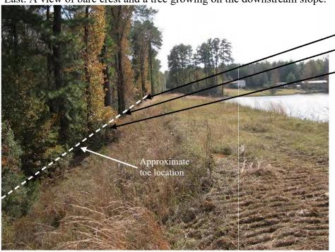
Photograph No. 6 – Standing near a midpoint looking North West. A view of the 3H:1V non-vegetated portion of the upstream slope and crest.
