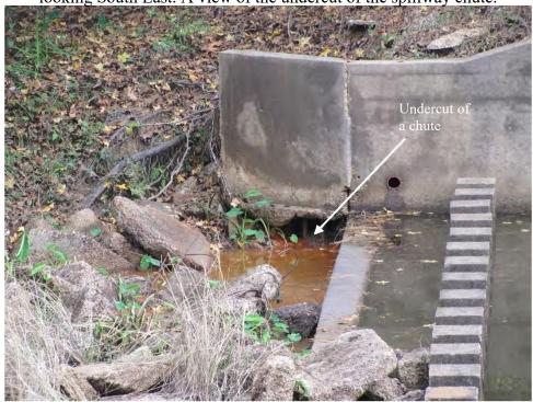
Photograph No. 46 – A view of the seepage on the right side of the downstream channel and undercut of the spillway chute.
