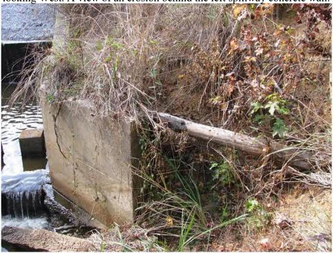
Photograph No. 44 – Standing just downstream of the spillway discharge looking North. A view of an undermined end wall (arrow).
