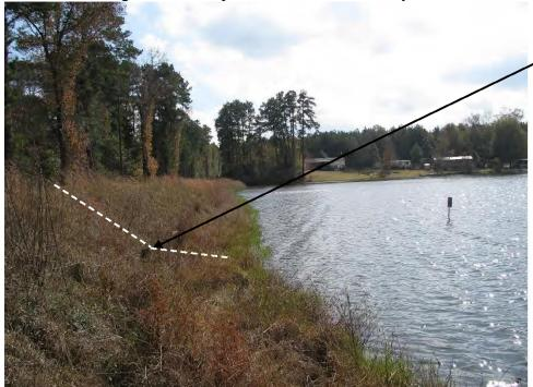
Photograph No. 10 – A view of the reservoir drain valve looking North East. A view of standing water standing and the toe erosion.
