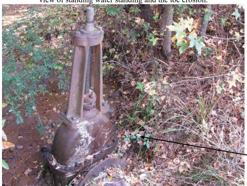
Erosion, as an indicator of high velocity turbulent flow
