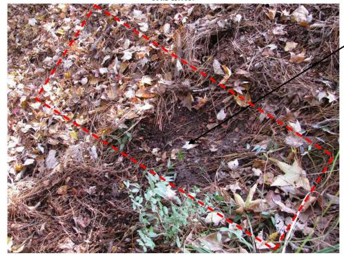
Seepage through the horizontal band 2 ft above the toe
