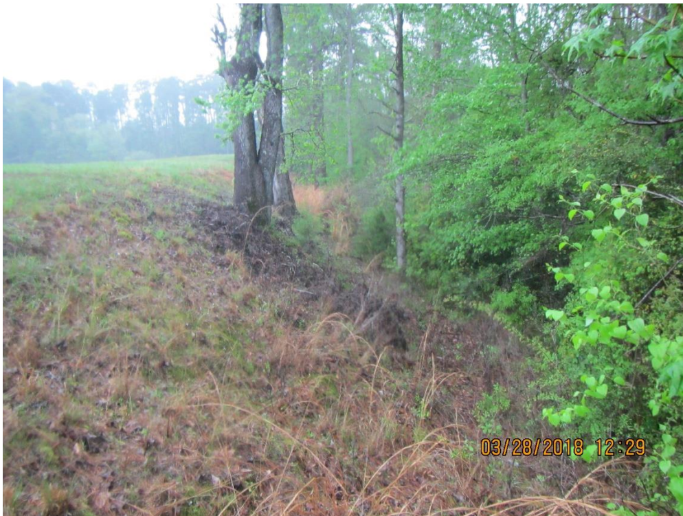
Photo 8: Standing on the right end of the dam looking northwest; a view of the large trees growing along the downstream slope.
