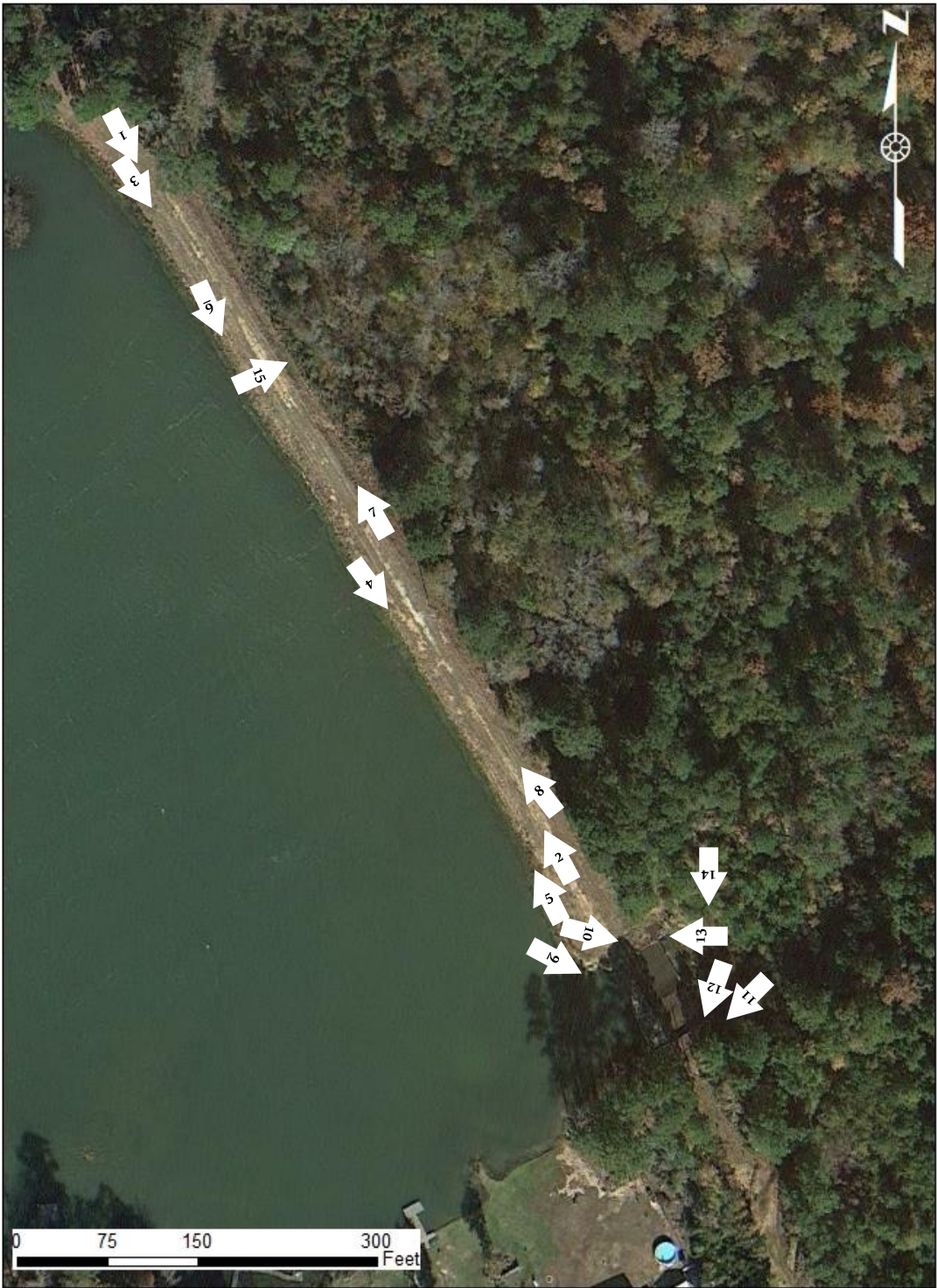
Figure 3 - Frog Pond Lake Dam TX03775 2014 Aerial View with Photo Locations
