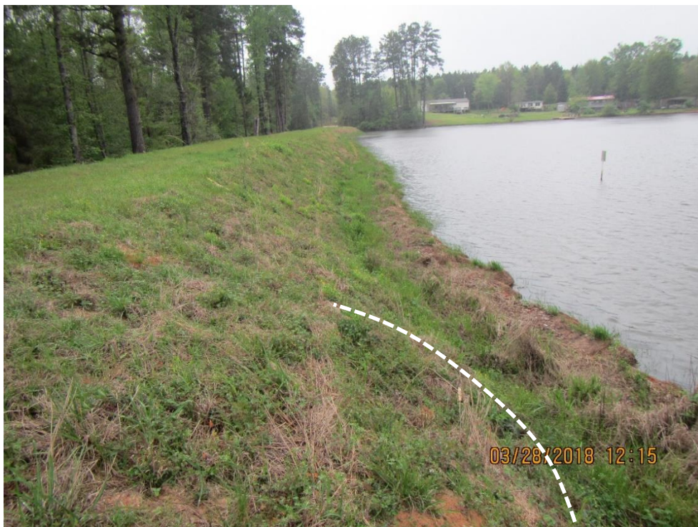
Photo 4: Standing near the midpoint of the dam looking southeast; a view of the 2H:1V vegetated portion of the upstream slope. Note the bulge near the midpoint of the dam (dashed-line).
