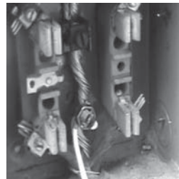
Step 2b Split-nut Installation
