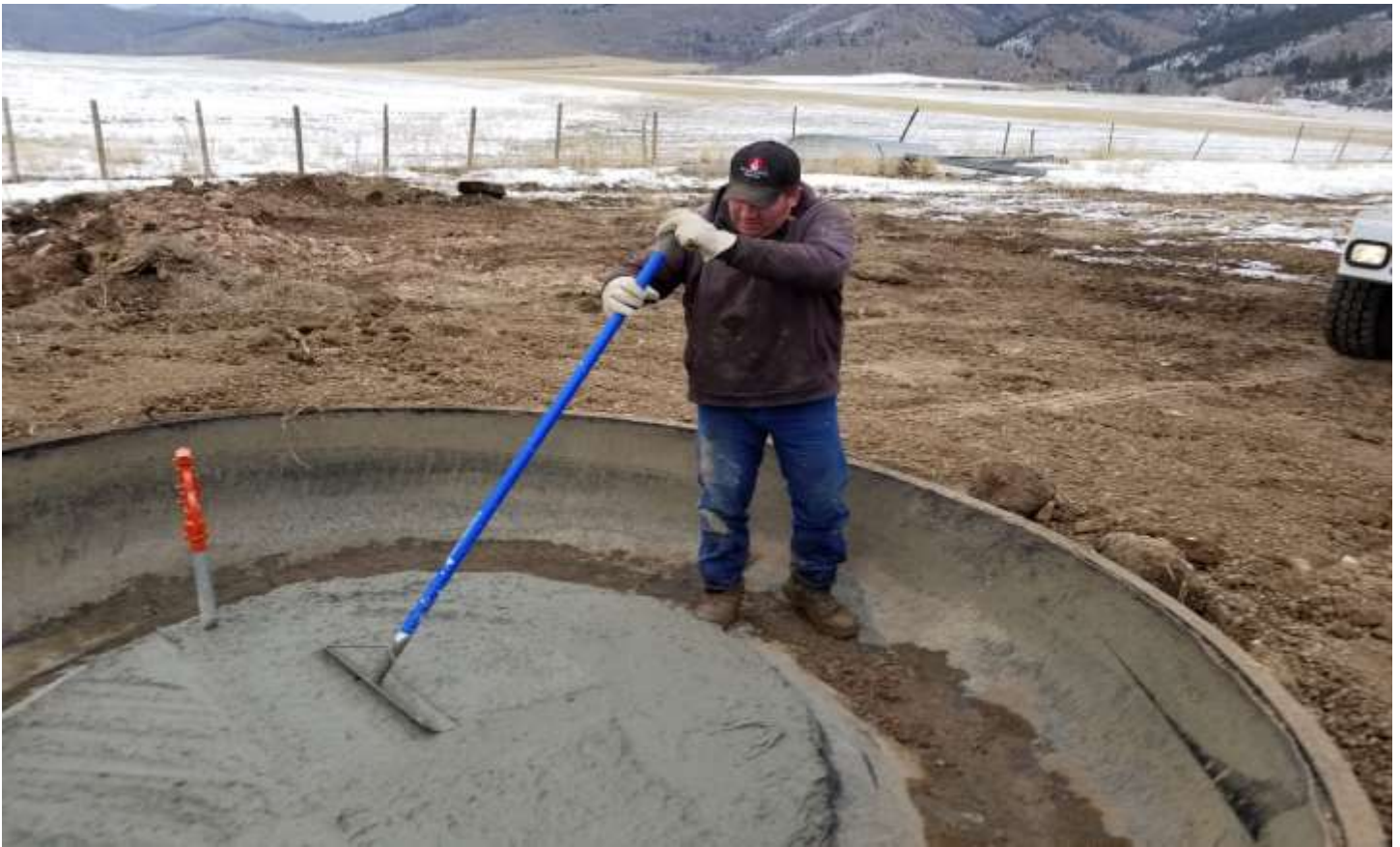
(Above) This photo shows the contractor putting the finish on the cement inside one of the troughs, SC Photos.
