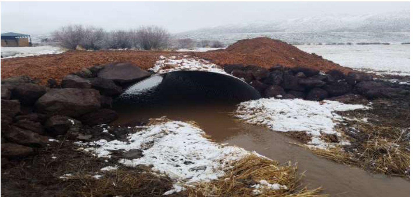
These two photos are the before and after of another stream crossing on Stauffer Creek. The historic culverts had washed out (one of two still pictured) and made it difficult for the landowner and for livestock to cross the stream. The lower photos shows the newly installed oversized culvert, which will provide access to the other side of the stream, and eliminate barriers to migrating BCT, SC Photos.
