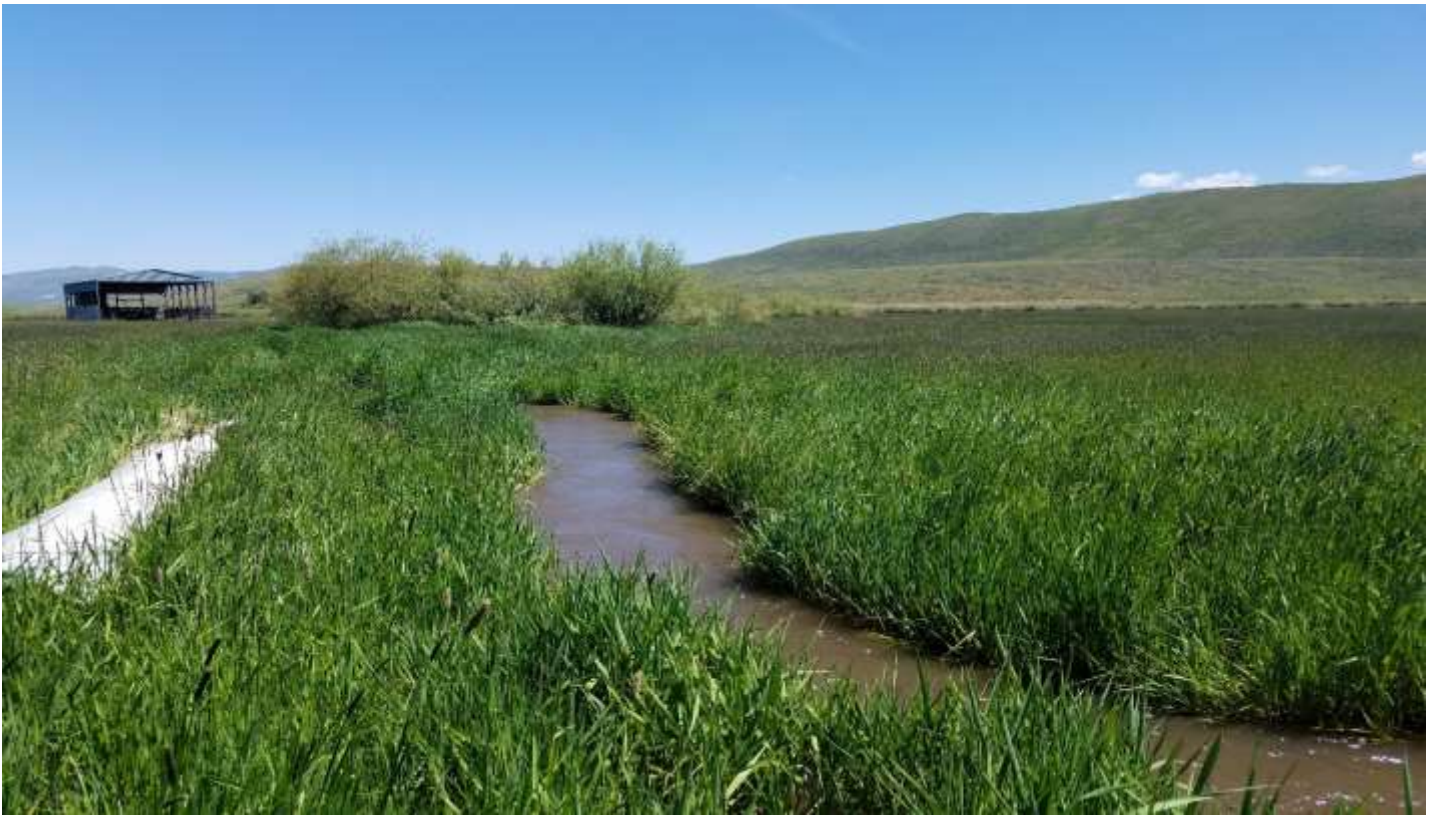
These two photos are the before and after of another stream crossing on Stauffer Creek. The historic culverts had washed out (one of two still pictured) and made it difficult for the landowner and for livestock to cross the stream. The lower photos shows the newly installed oversized culvert, which will provide access to the other side of the stream, and eliminate barriers to migrating BCT, SC Photos.
