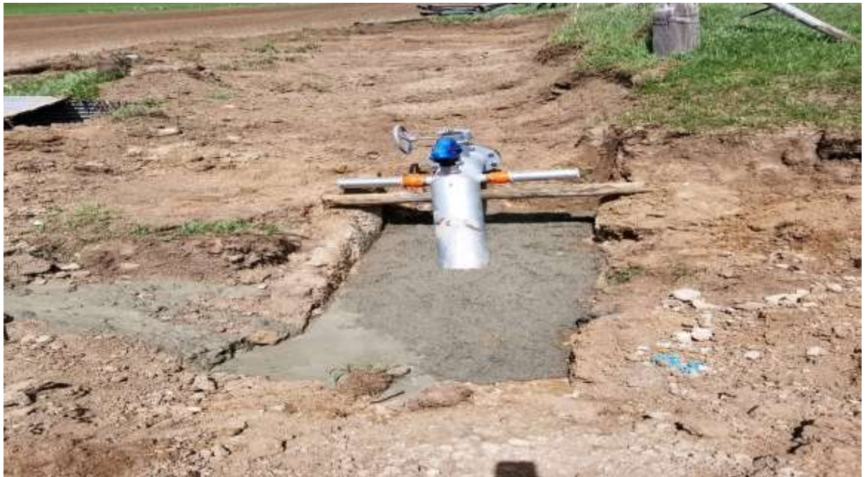
The above photo shows the end of one of the sections of mainline after it was installed. It was prepped for a thrust block to be poured to hold it in place. The lower photo shows the same pipeline after the thrust block was poured. BLD Photos.
