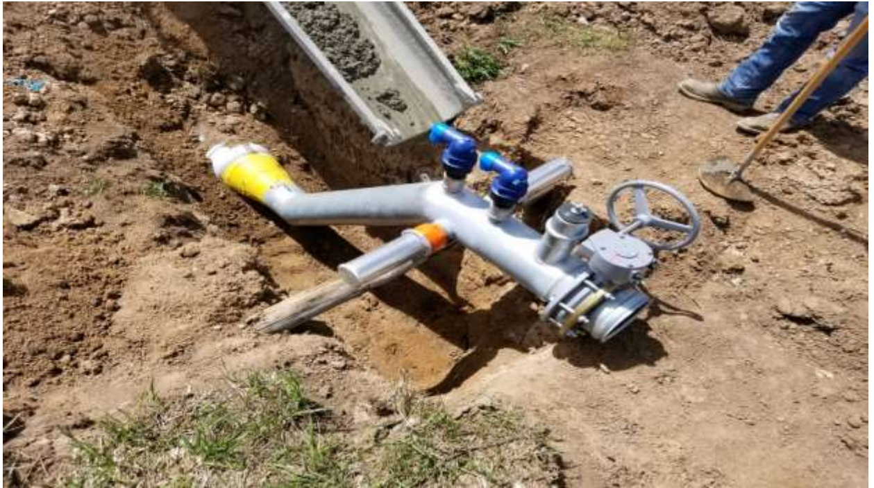
The above photo shows the end of one of the sections of mainline after it was installed. It was prepped for a thrust block to be poured to hold it in place. The lower photo shows the same pipeline after the thrust block was poured. BLD Photos.
