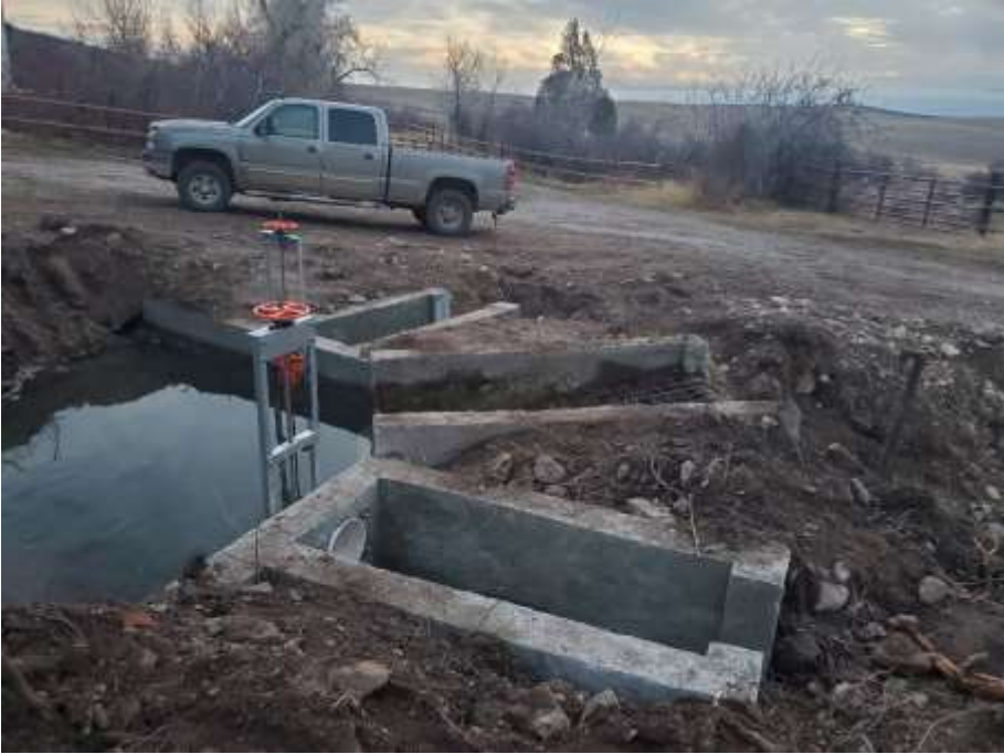
Both of these photos show the bennington diversion. The upper photo is the old diversion before implementation. The lower photo shows the newly installed diversion structure. BLD photos.
