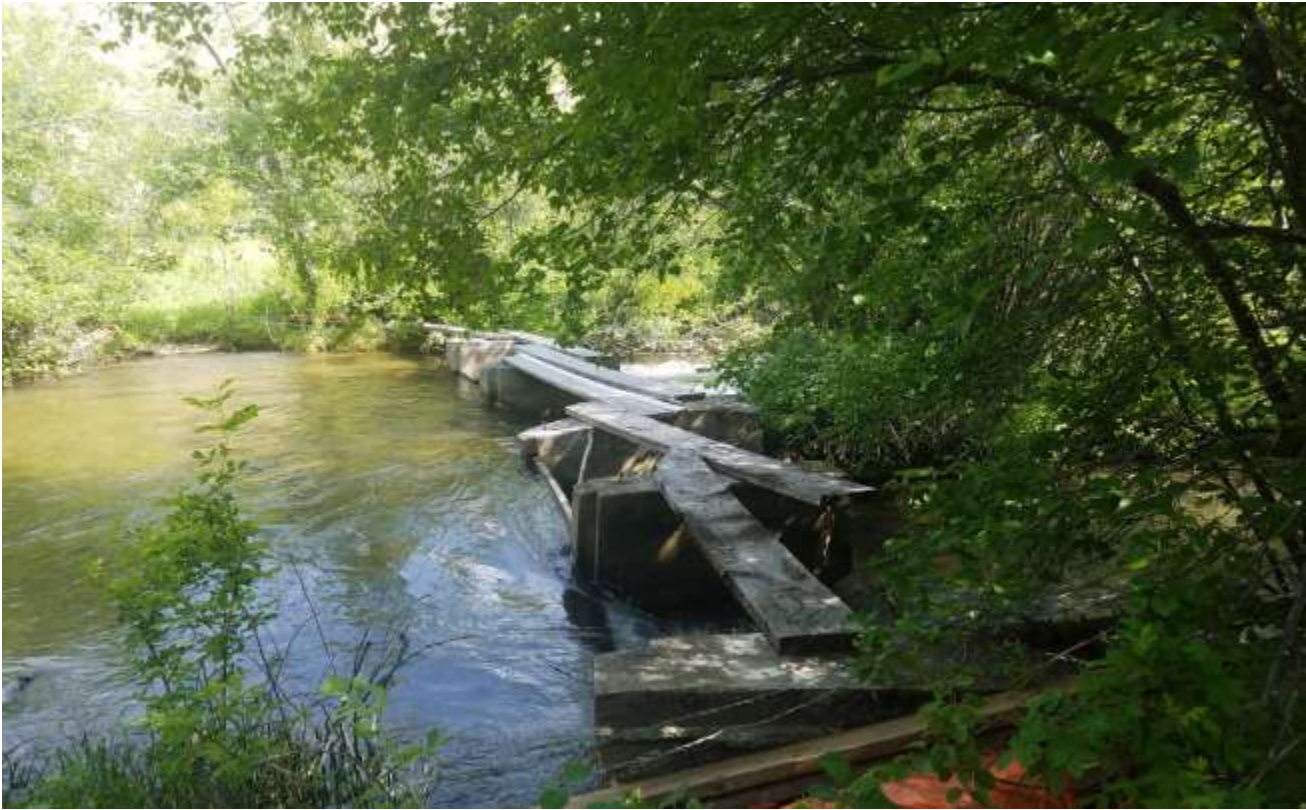
The photos on this page show the St Charles Diversion Structure in St Charles Creek. The above photo shows the dilapidated old structure. The old diversion was about one large runoff event from washing downstream. The lower photo shows the newly installed diversion structure. Both photos show the diversion from South to North BLD Photos.
