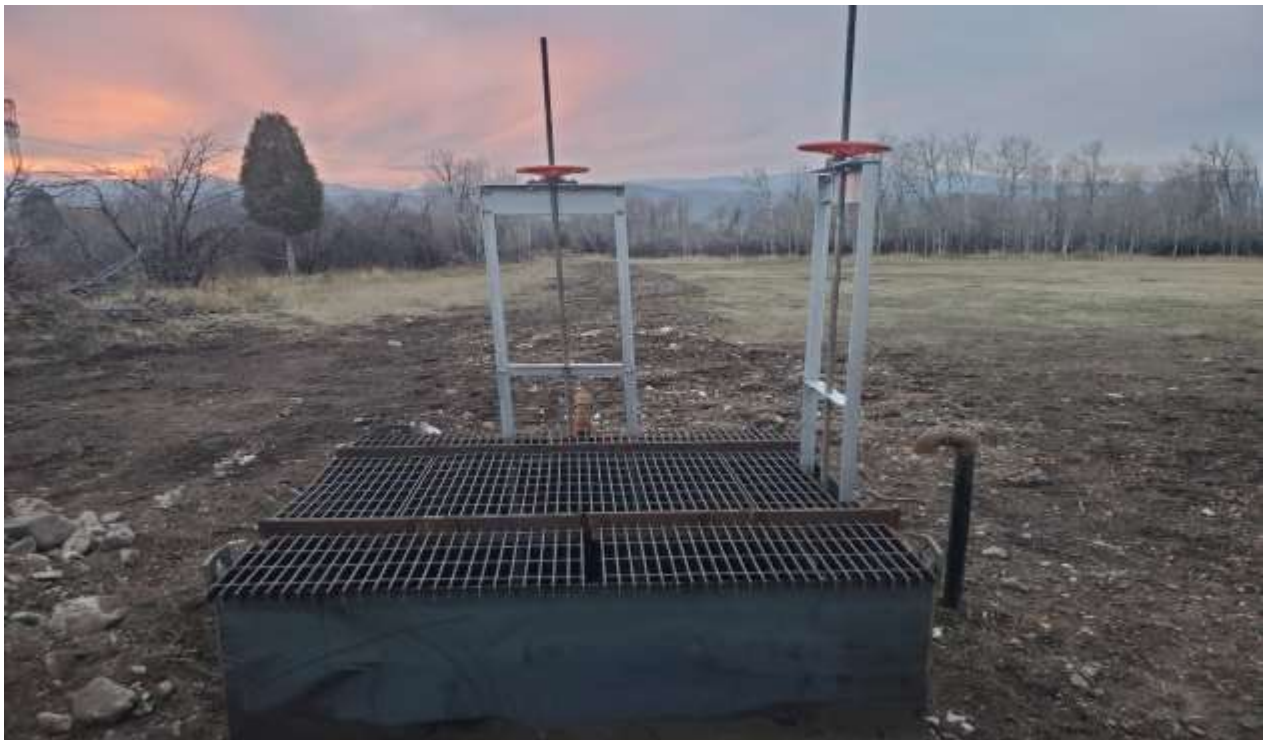
The upper photo shows what the two smaller sides of the bennington Diversion look like. These two side diversions are made to handle smaller amounts of water. The Bottom photo shows the junction box which splits water from the trunk line and sends it two different directions. BLD Photos.
