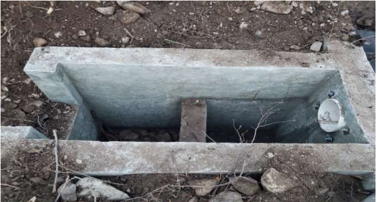
The upper photo shows what the two smaller sides of the bennington Diversion look like. These two side diversions are made to handle smaller amounts of water. The Bottom photo shows the junction box which splits water from the trunk line and sends it two different directions. BLD Photos.
