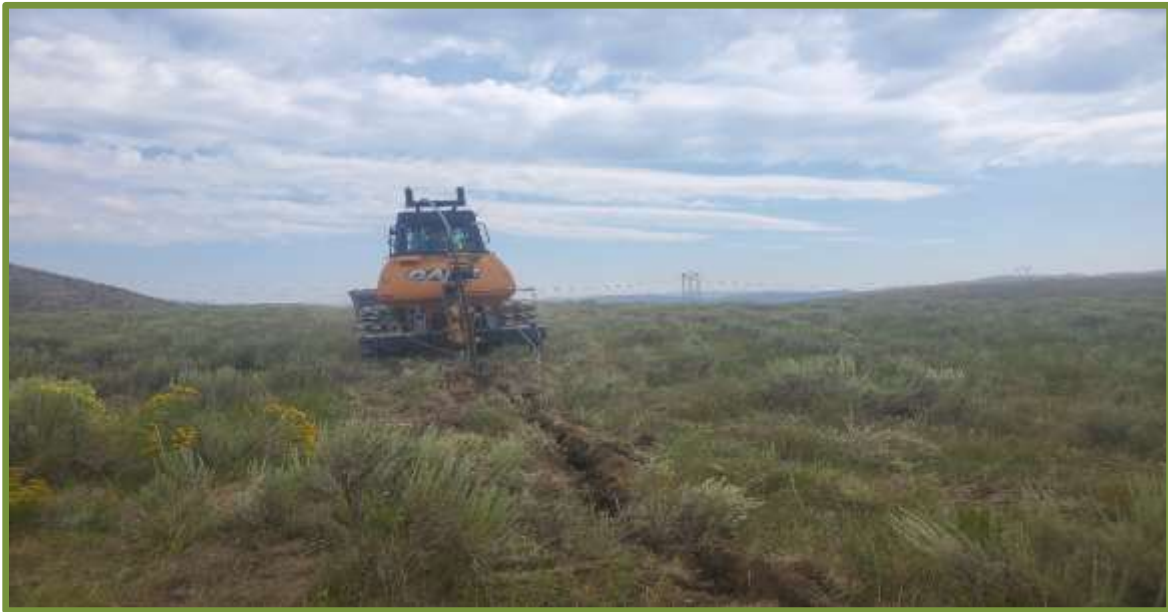
Pipe being ripped in during installation of one of the Stockwater systems for Chesterfield Land and Livestock, UBR Photos.
