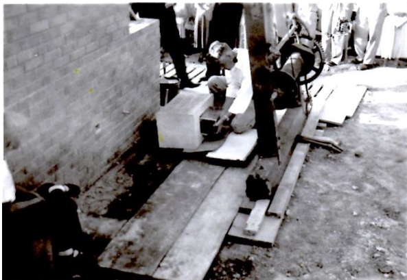
Laying of the corner stone
