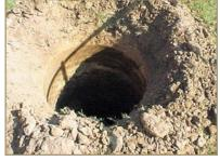
The hole diameter selected for the embedment should allow a minimum clearance around the corners of the pole butt of 4 to 6 inches. Hole sizes are generally specified in 6 inch increments to accommodate standard auger sizes. The hole diameter for octagonal poles may be determined by adding 8 to 12 inches to the width of the pole butt.
