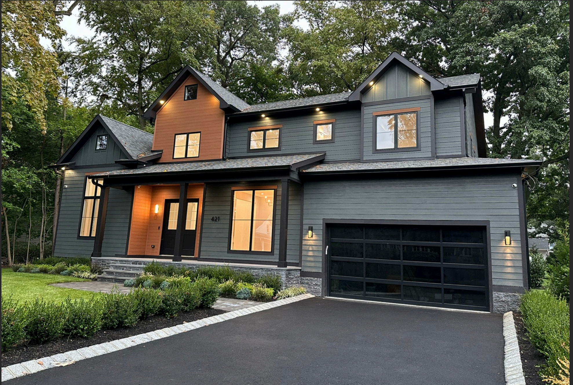
421 Sylvan Pl at dusk. Hardie siding in Iron Gray along with Nichiha siding as an accent
