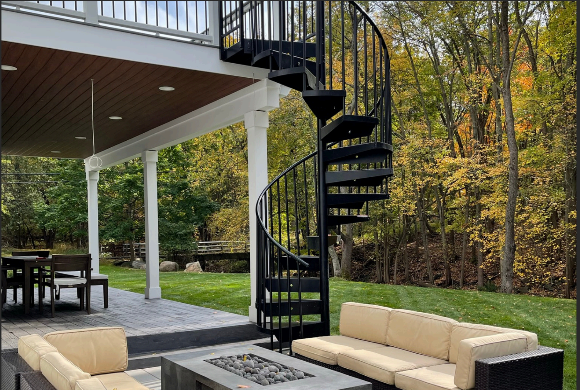
Spiral staircase made with powder coated aluminum leading to a Trex deck above. Outdoor patio with natural gas fireplace in concrete.
