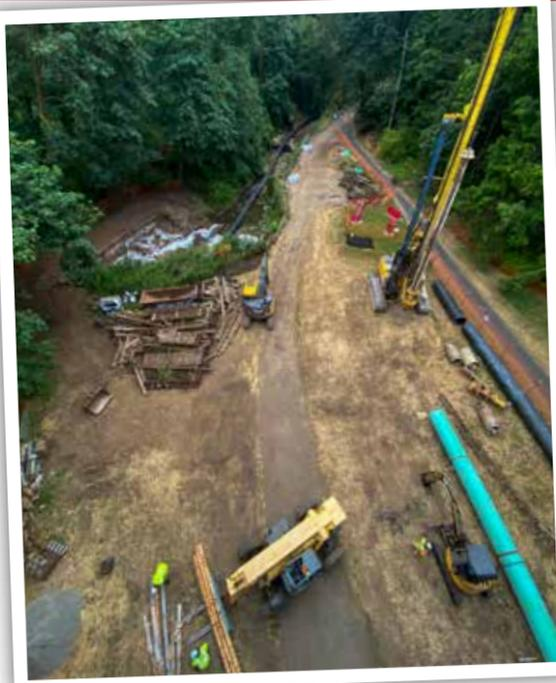
The Bureau of Development Services is replacing the wooden trash rack over Balch Creek in Lower Macleay Park, where the stream is diverted into a culvert that empties into the Willamette River. Photo by Matt Erceg
