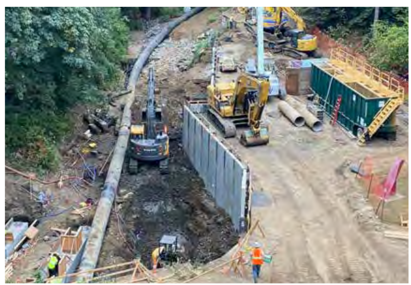
Work continues on replacement of the Balch Creek trash rack in Lower Macleay Park. Lower Macleay Trail will remain closed until the project is finished, projected to be by the end of the year. Photo by Scott Kocher
