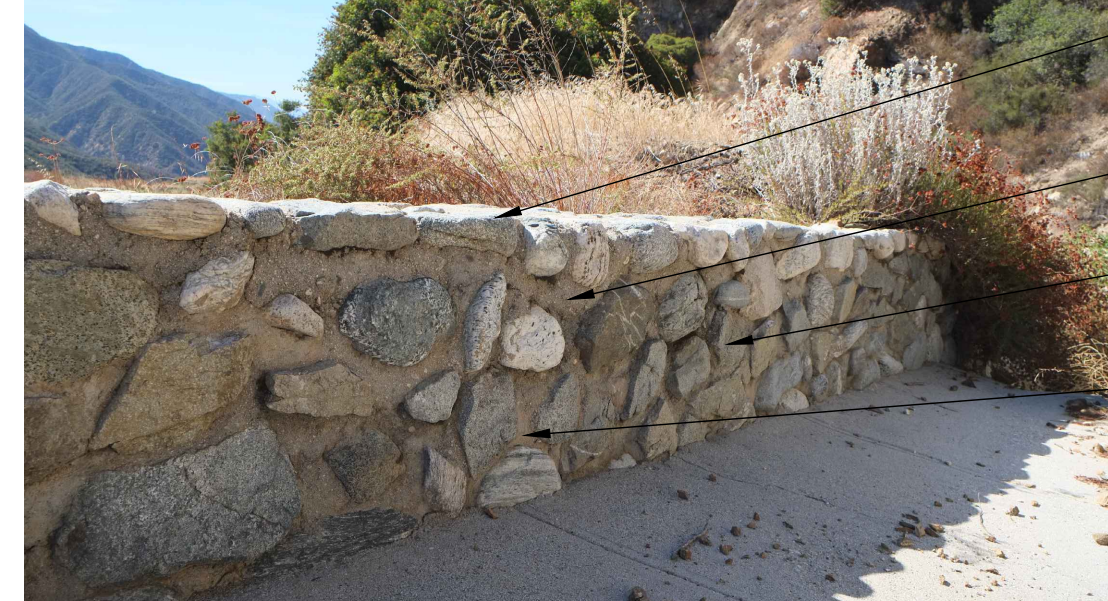
SAMPLE ROCK BARRIER WALL NEAR PROJECT SITE
