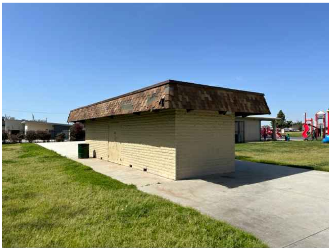
EXISTING RESTROOM & ELECTRICAL ROOM BUILDING
