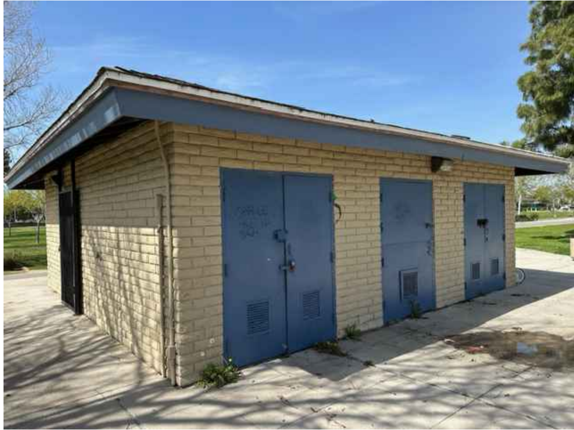
EXISTING RESTROOM BUILDING
