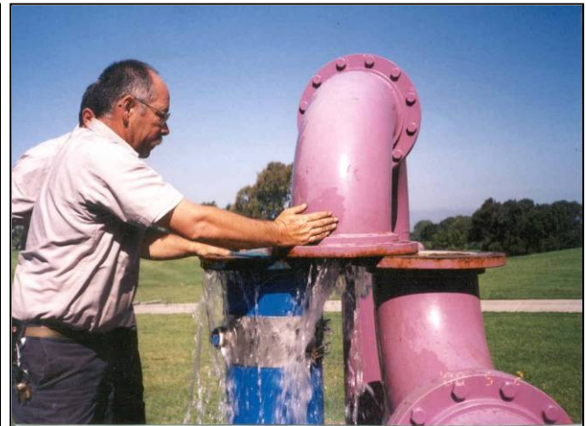
Example photos of existing "swivel-ell" assemblies for a back-up potable water supply.
