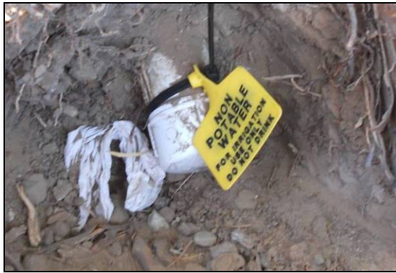
Non-potable water identification tag (yellow)
