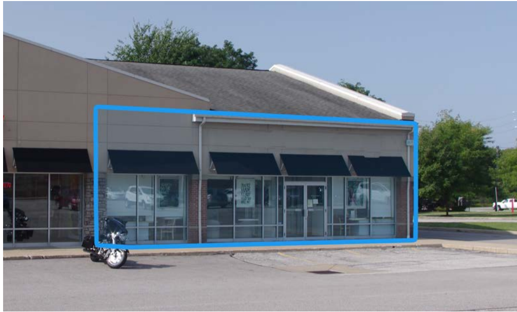
3,080 SF bank location
