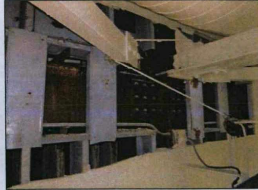
Photo 14. Intermediate column-beam connection at Location 6.
