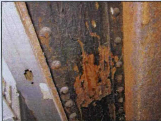
Photo 1. Coal tar coating on column at Location 1.
