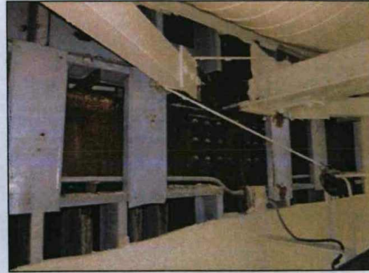
Photo 14. Intermediate column-beam connection at Location 6.
