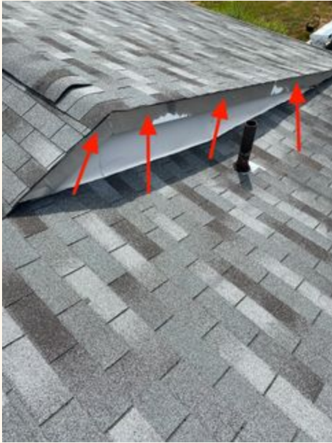
The flashing has lost its exterior paint and is susceptible to an increased rate of deterioration.
