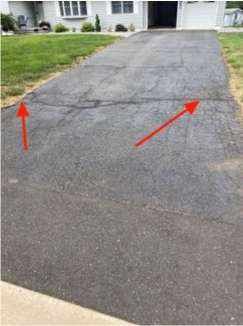
Cracks were noted in driveway flatwork. Repair as needed.
