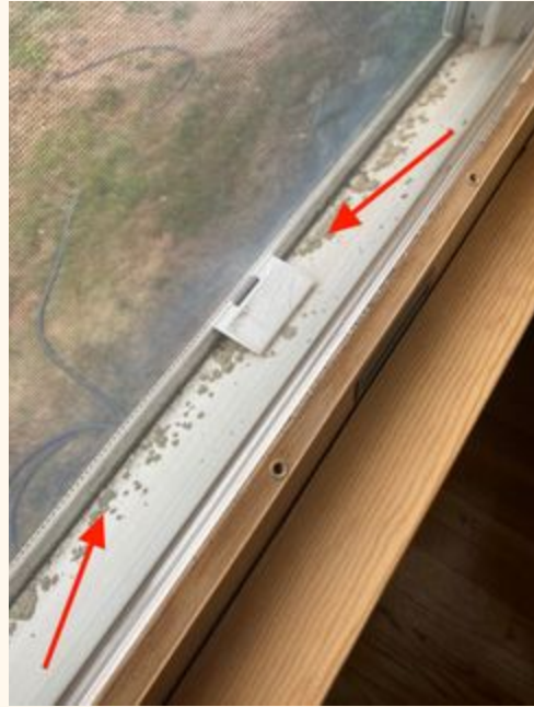
Mold-like growth found on south facing windows of new master bedroom
