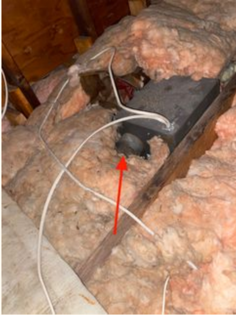
Bathroom fan is not venting out to the exterior.
