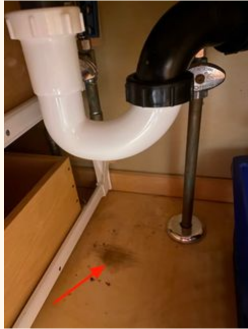
Leak causing water damage to the interior base of the vanity.
