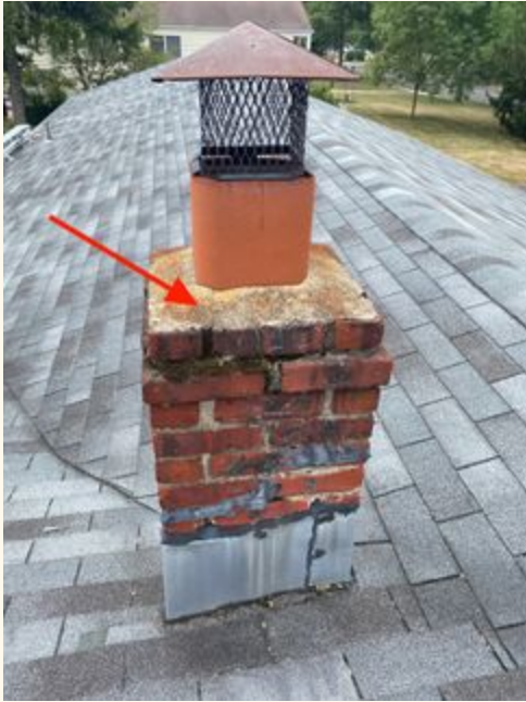
Arrow indicating the cement wash chimney crown. It is recommended for the chimney crown to overhang the chimney stack by two inches to prevent deteriorating of the chimney stack.
