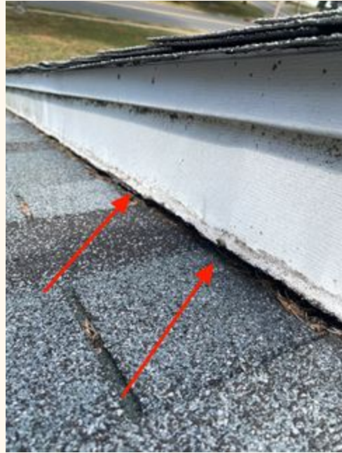
Minor lifting of this flashing where the garage roof and house roof meet.
