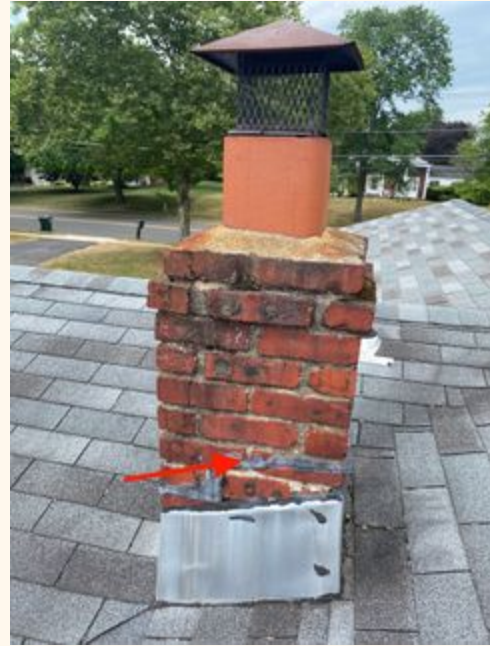
Around the chimney mortar, sealant was used. This is not a proper way to seal the chimney and it is recommended for a qualified mason to further evaluate and make repairs.
