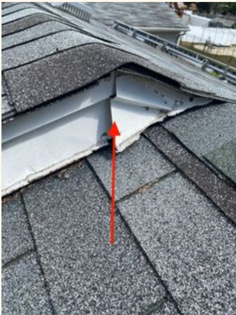
Flashing pulling away at the ridge of the roof.
