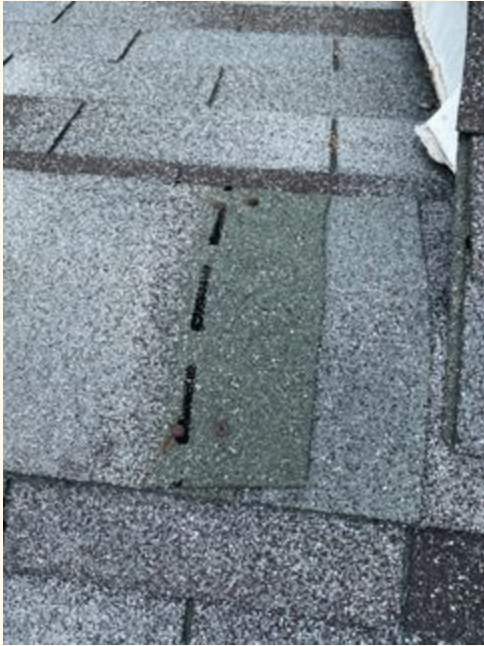
Arrows indicating the nails that are unsealed which can allow for water intrusion.
