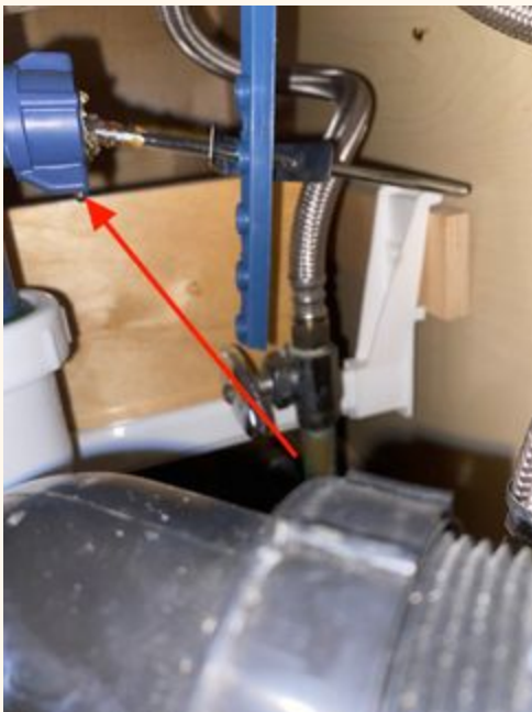
Location of the leak is coming the the sink stopper mechanism.
