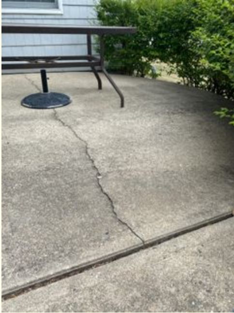
Arrows are pointing at the large crack through the concrete slab.
