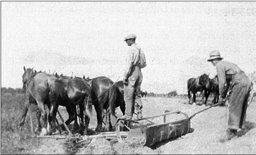
Road Construction in the early 30's
