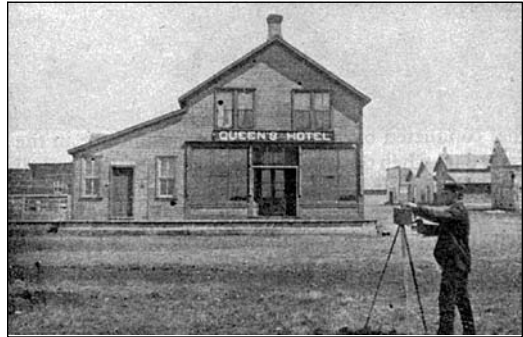
Queen's Hotel - site of first meeting of the local improvement district.
