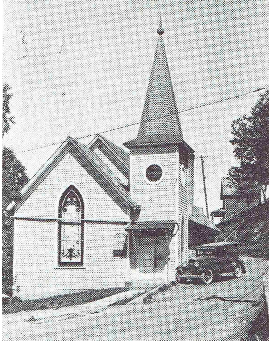
The first building of the Scandinavian Lutheran Church of Lead (later called Bethel Lutheran Church) on the corner of Wall and Addie Streets in Lead.
