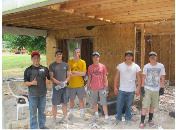
The youth helped to tear down this house damaged by Hurricane Florence.
