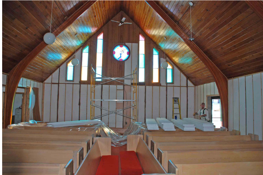
The paneling was removed from the sanctuary in 2009. It was replaced by insulation and finished sheet rock.
