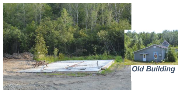
Slab for New Building
