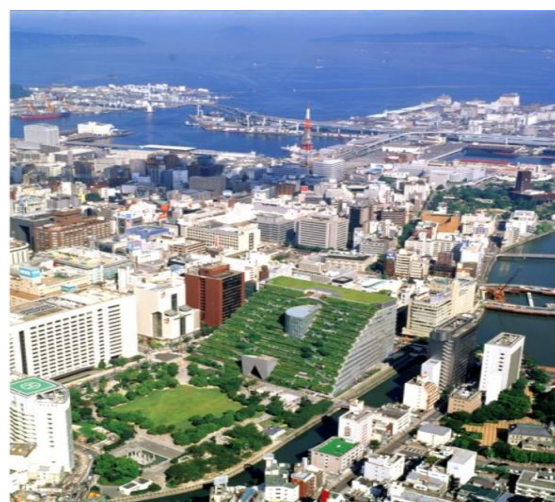
Figure 2. The ACROS Building (Velazquez, 2011).
