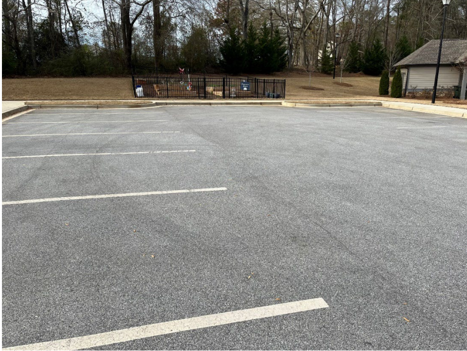
1. View of amenity area parking lot.
