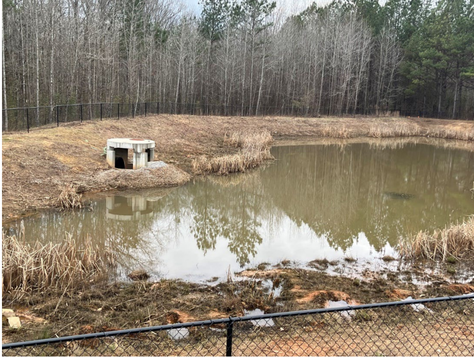
11. View of retention pond.
