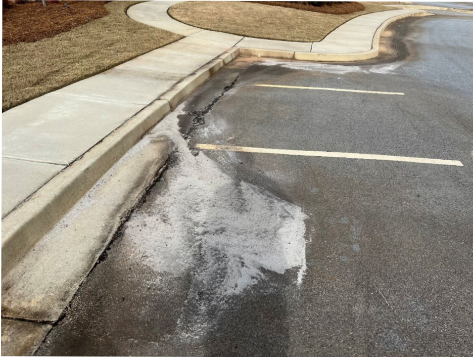
9. View of area with accumulated sediment near tennis court and pavilion
