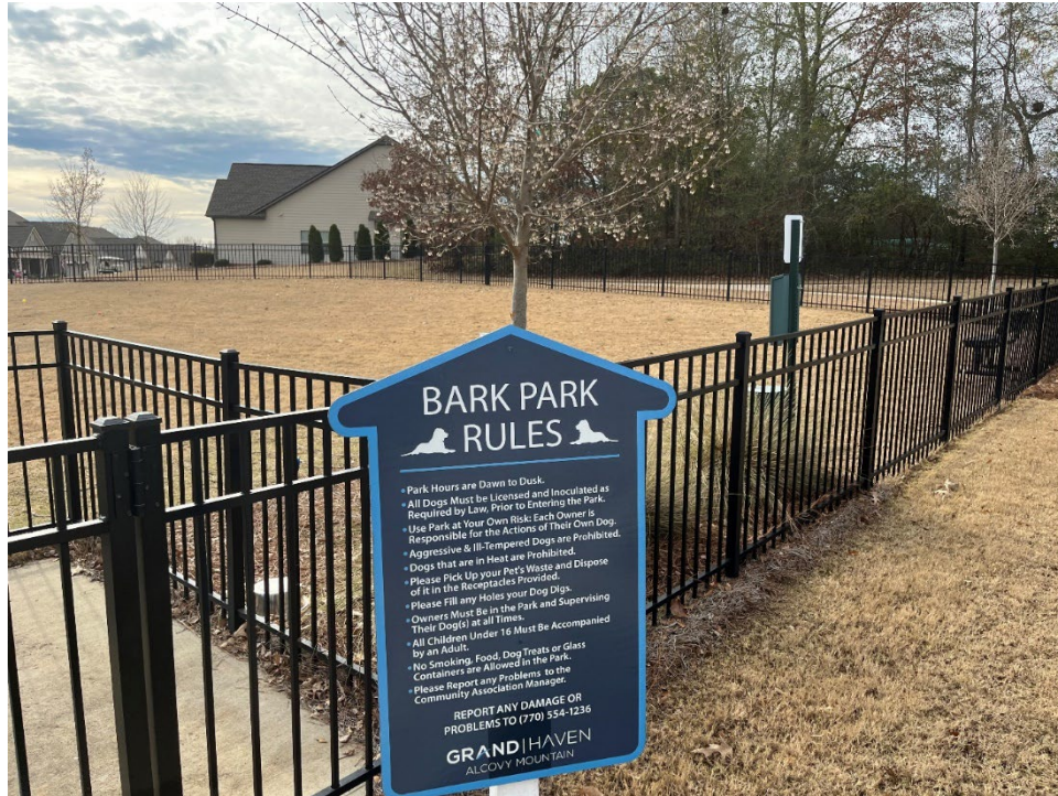
7. View of aluminum fencing at dog park.
