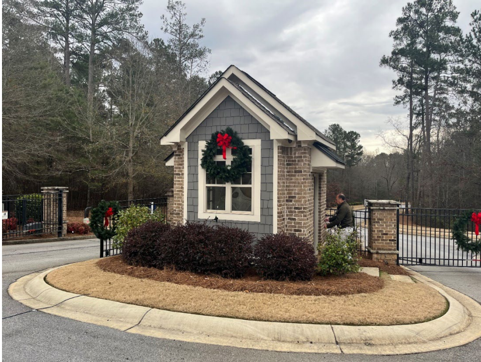
29. View of guardhouse and entry gates.
