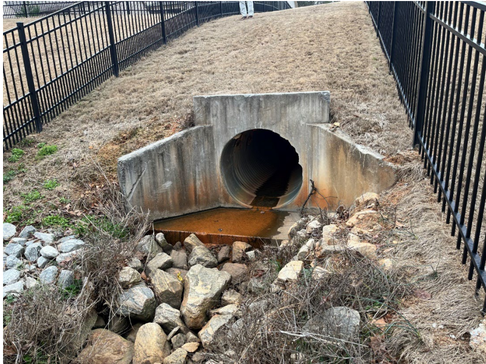
8. View of typical community drainage system.
