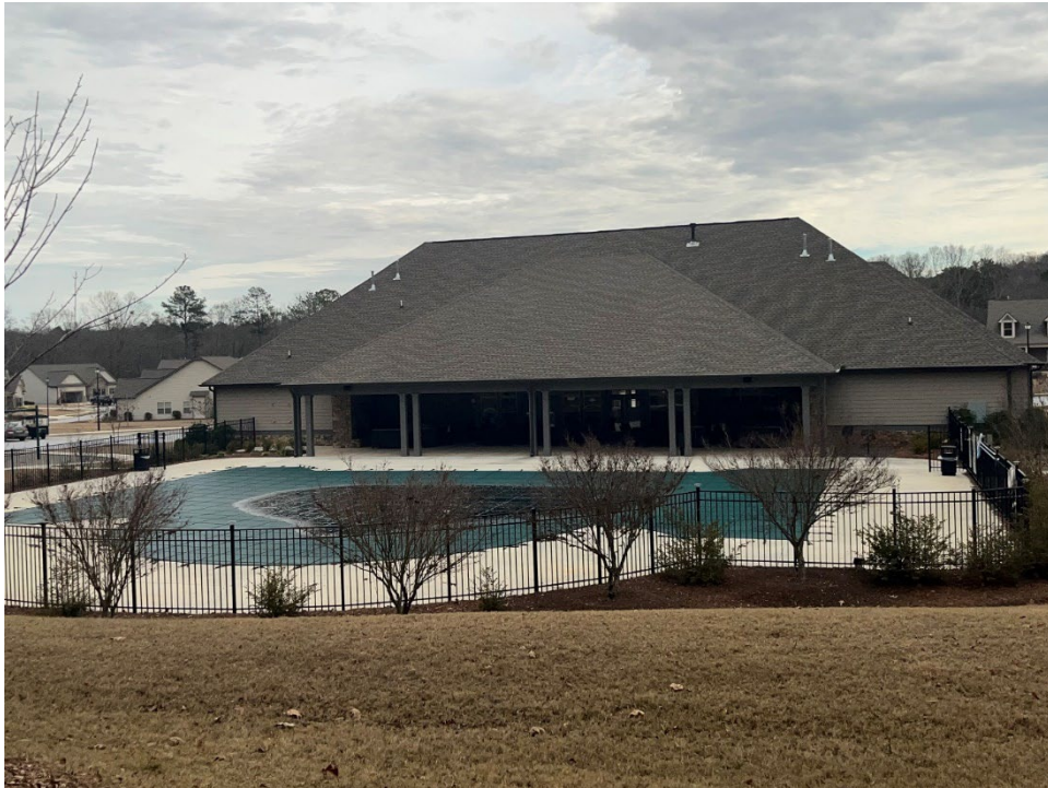
22. Rear view of clubhouse.
