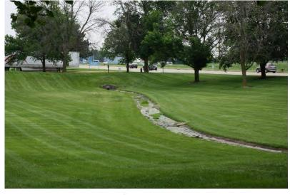
Typical Dry Bottom Turf w/Channel
