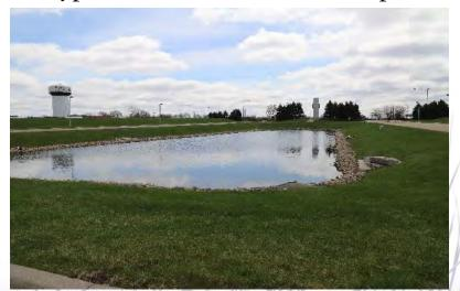
Typical Wet Bottom-Riprap Slope
