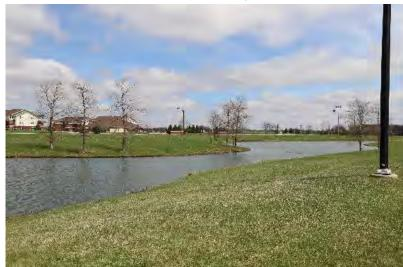
Typical Wet Bottom-Turf Slopes
