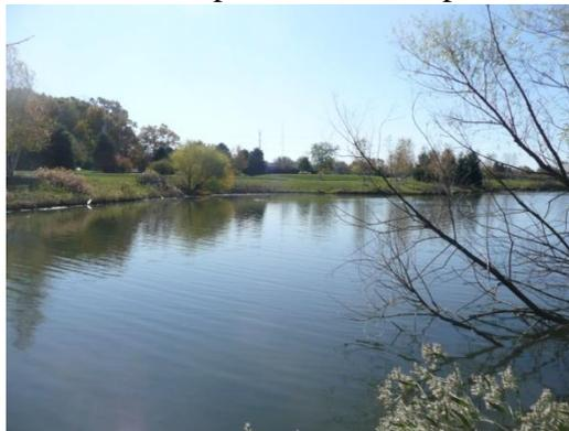
pollutants such as sediments to settle to the bottom of the basin. In addition, wetland vegetation helps to filter out pollutants and utilizes others, such as fertilizers, as storm water passes through the basin.
