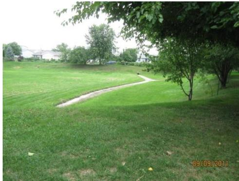
Detention basins detain water and are designed to be dry between rain events. During a storm they fill with storm water. These basins slow the rate at which storm water from new developments enters the streams and rivers and thus helps prevent
